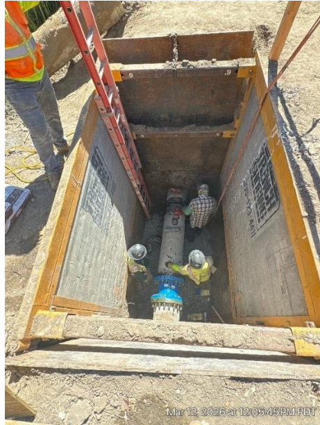
Phase 2 Pipe Connection at Receiving Pit
