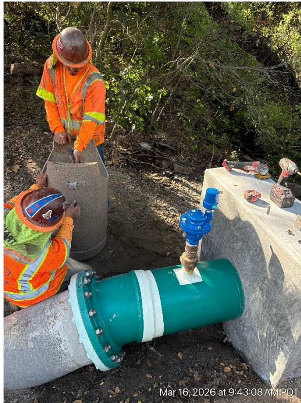
Phase 1B Air-Vac Installation
