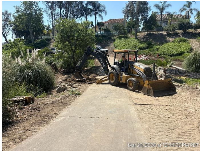
Phase 2 Receiving Pit
