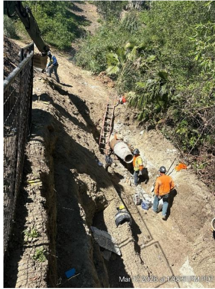
Phase 2 Installation of Reducer
