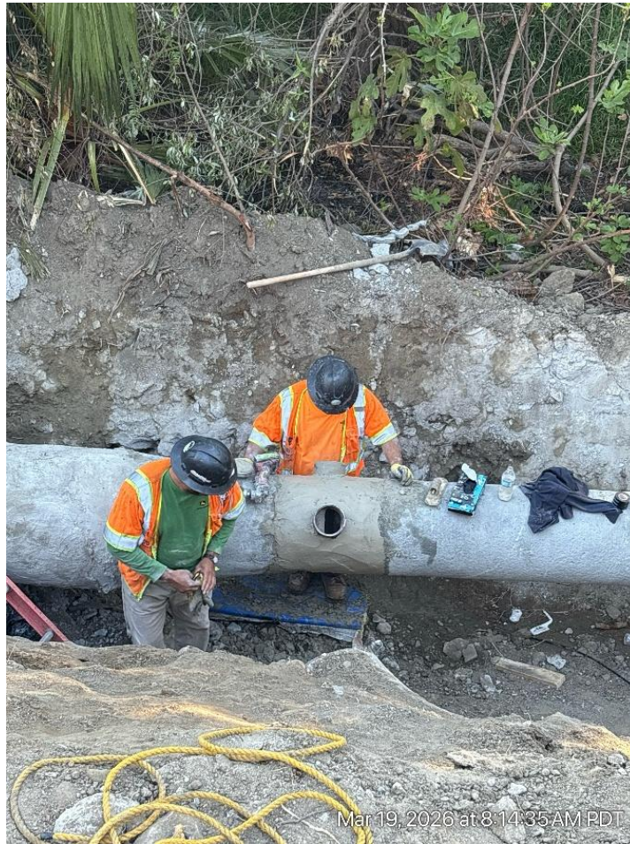
Grouting of Hand-Hole
