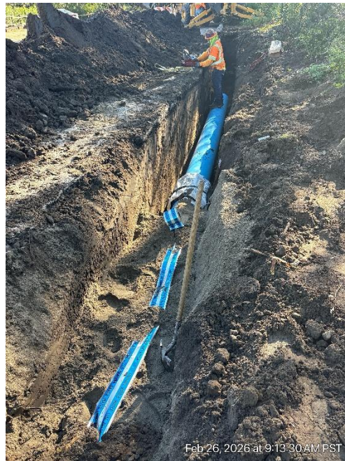
Open Cut Pipeline Installation
