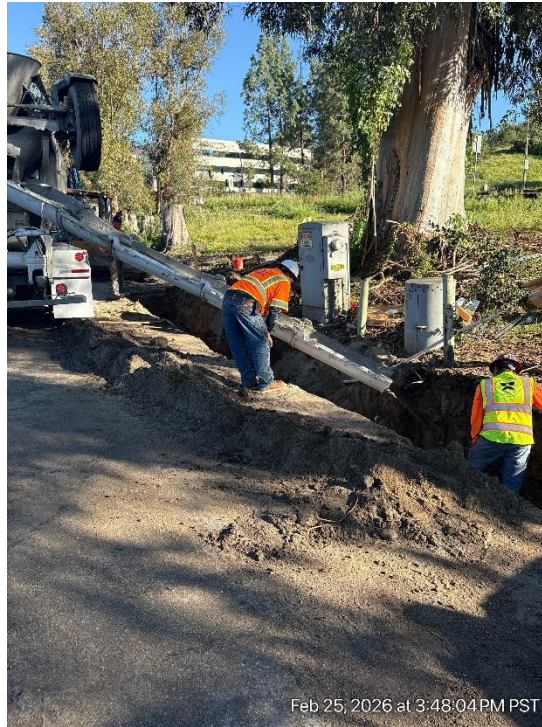
Placement of Thrust Block
