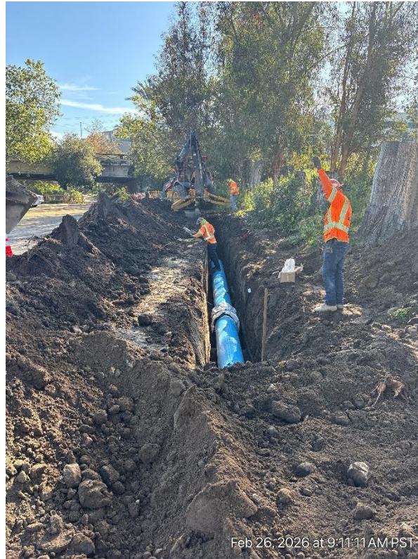
Open Cut Pipeline Installation
