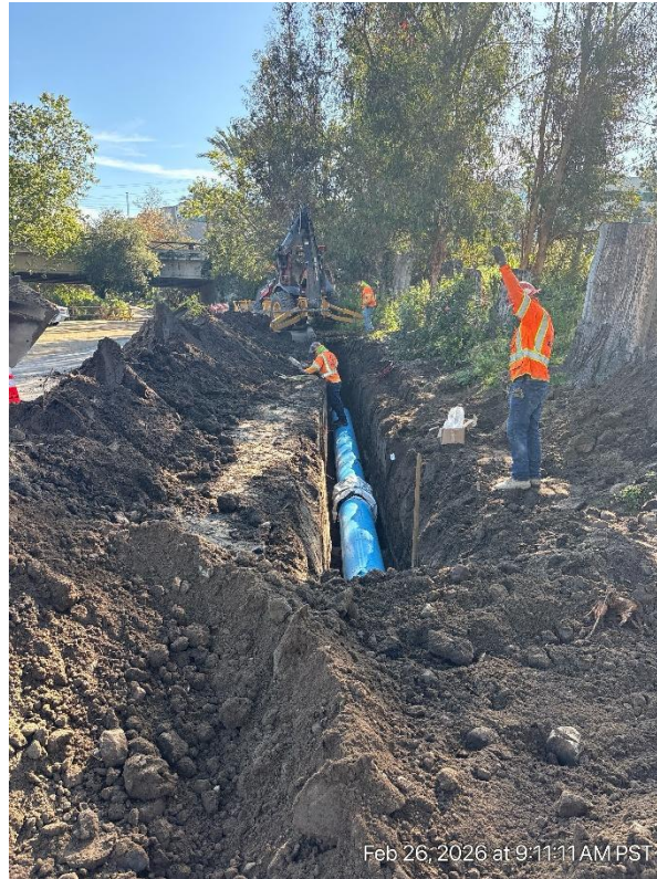
Open Cut Pipeline Installation
