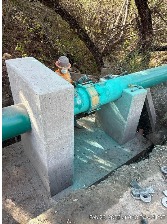
Creek Crossing Pipeline Installation
