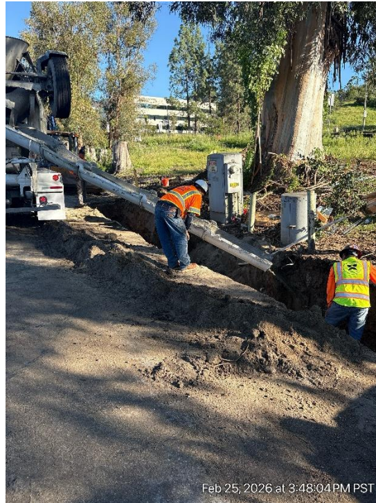
Placement of Thrust Block
