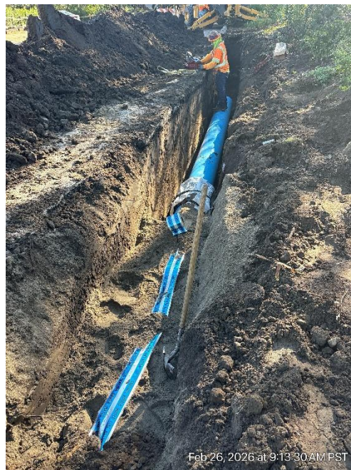
Open Cut Pipeline Installation
