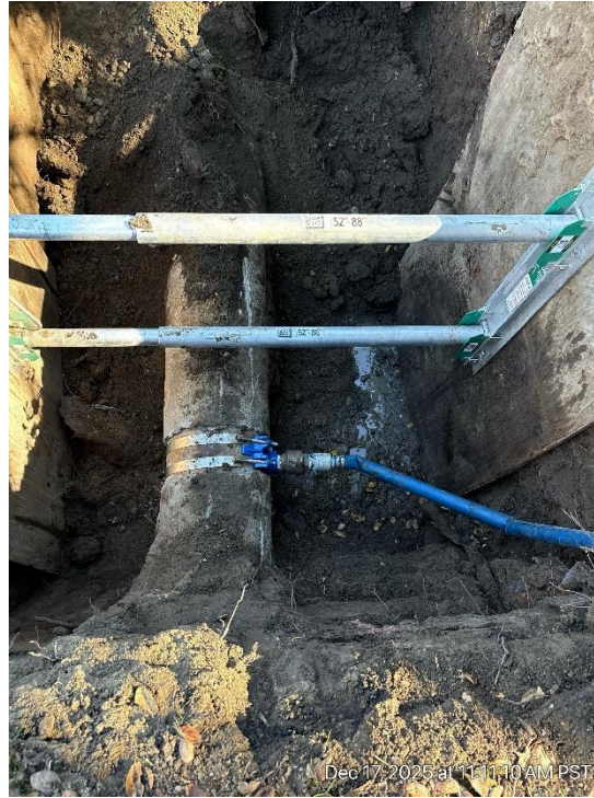
Hot Tap to drain excess water
