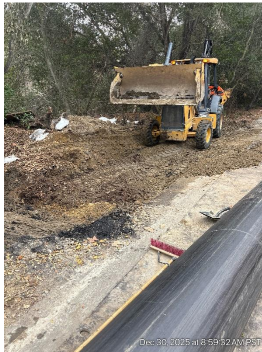
Pit Backfill
