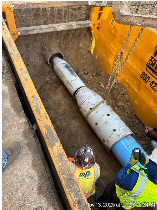
Insertion of Pipe Bursting Head
