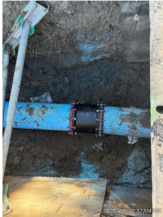
Coupler Connection of C900 Piping After Pipe Bursting
