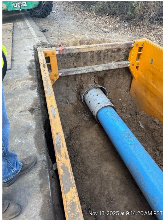
Began Pipe Bursting
