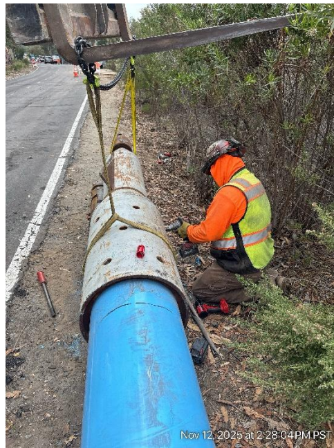
Installed Pipe Bursting Head
