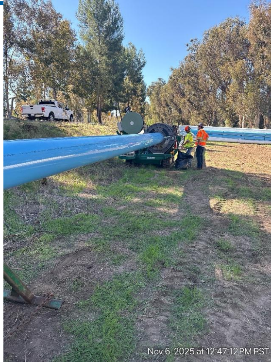
Fusing C900 Piping
