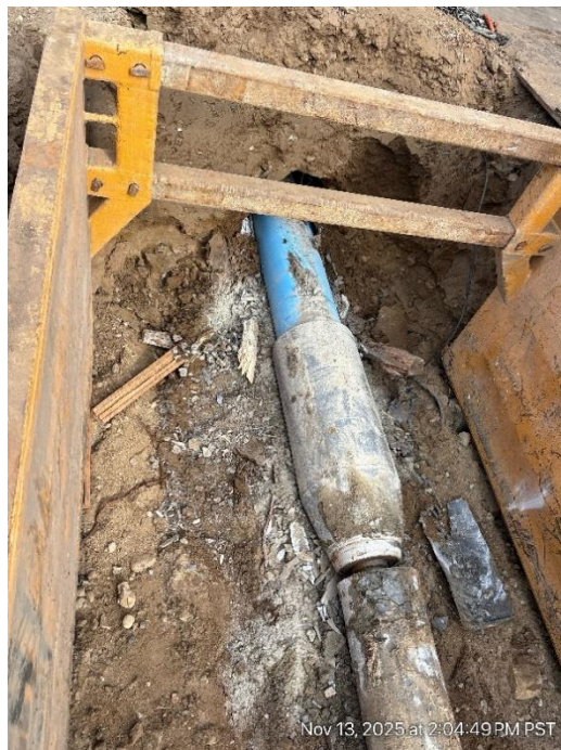
Completed Pipe Bursting
