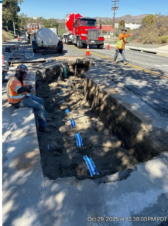
PIPE-ZONE SAND BACKFILL WITH WARNING TAPE
