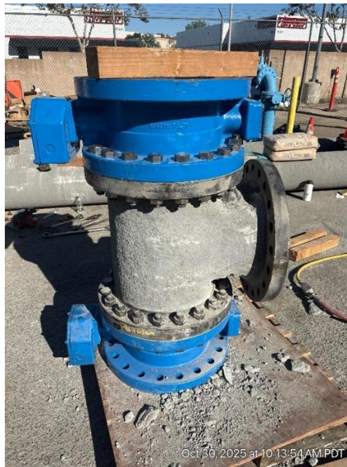
FIT UP OF VALVES TO THE T-FITTING FOR PIT #1
