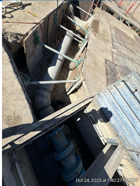
PIPING INSTALLATION FROM THE PIPE VAULT TO PIT #1
