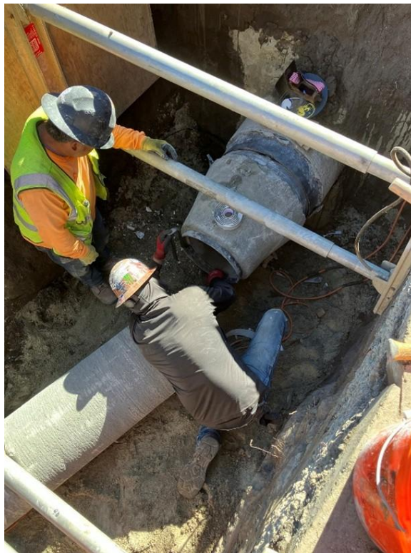
PIPING INSTALLATION IN PIT #3
