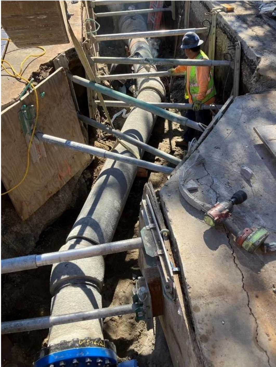
HARD-PIPING INSTALLATION IN PIT #3
