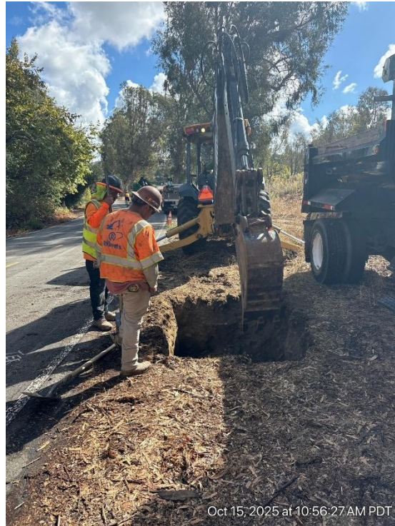
PHASE 1B POTHOLING
