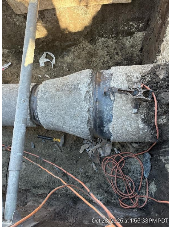
INSTALLED 24" X 16" REDUCER AT PIT #3
