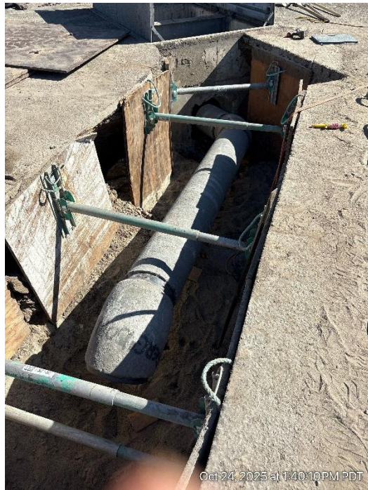
PIPING INSTALLATION FROM THE EXISTING VALVE VAULT TO PIT #1
