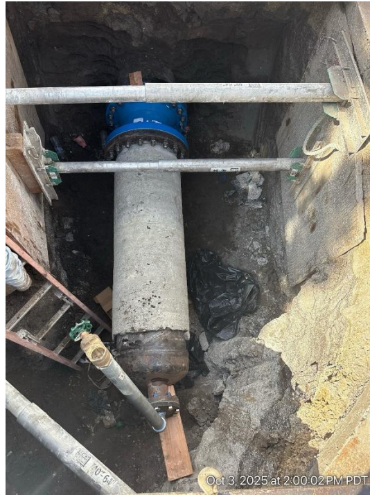
PRESSURE TESTING BETWEEN PIT #1 TO PIT #3
