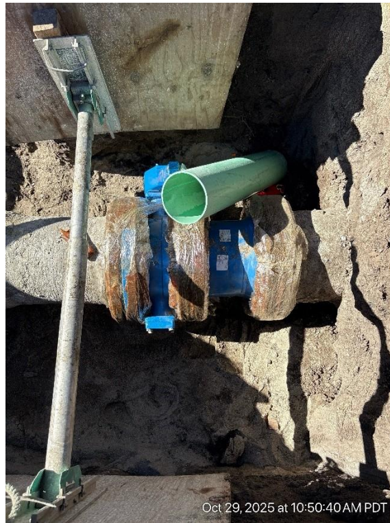
VALVE INSTALLATION IN PIT #3
