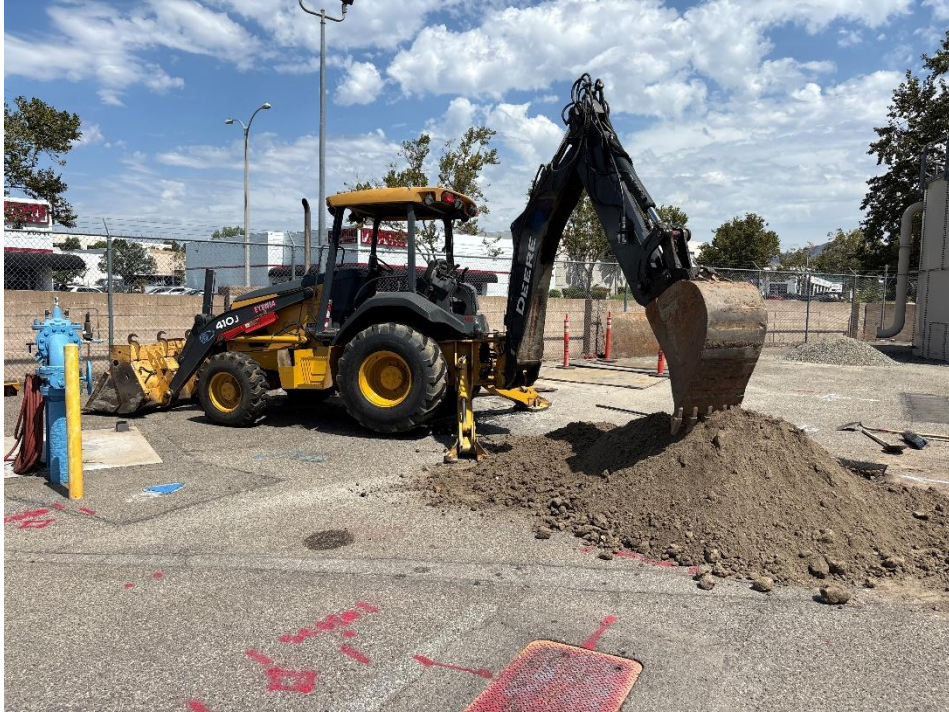
EXCAVATING PIT #1 AT DIMENSION WATER TREATMENT PLANT
