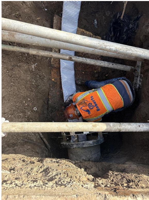
INSTALLING PRIMUS LINER
