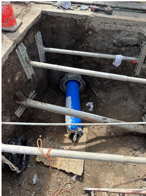
Inflating Primus Liner with Air Compression
