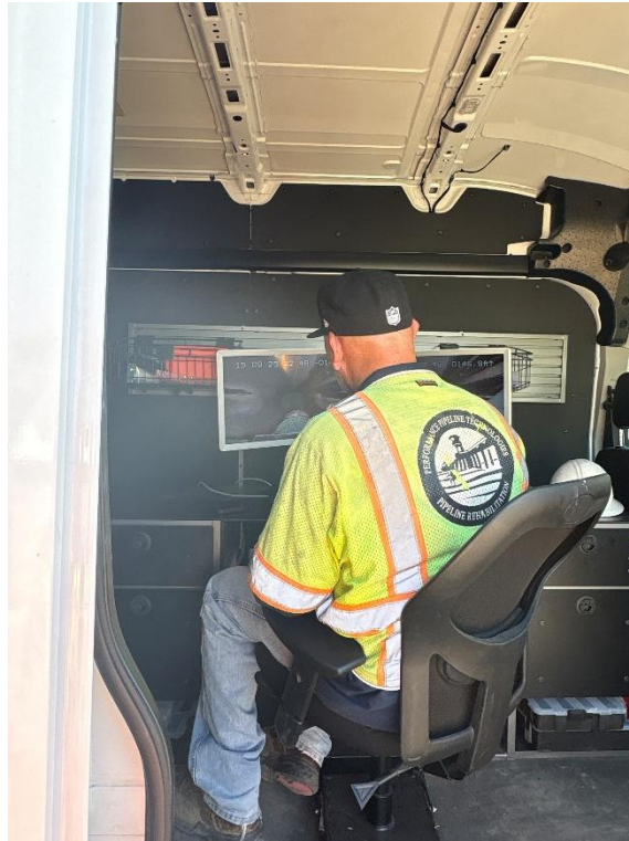
PIPELINE INVESTIGATION AND PIPE CLEANING
