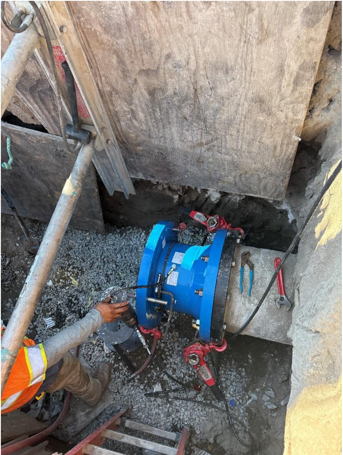
HIGH PRESSURE INJECTION OF RESIN INTO R-CONNECTOR FITTING
