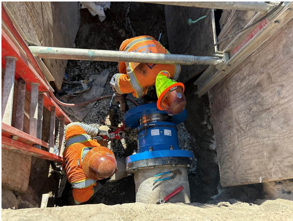
Installing Primus R-Connector Flange Fitting
