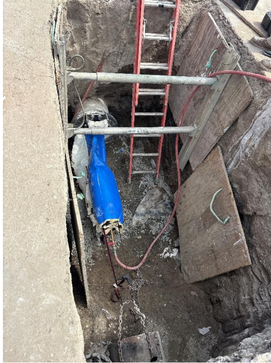
Inflating Primus Liner with Air Compression
