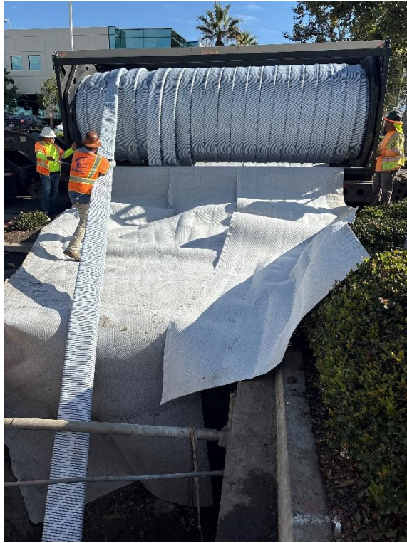
INSTALLING PRIMUS LINER
