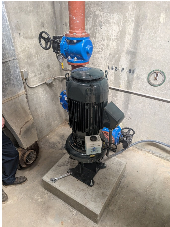
TCWD Operations delivered and installed Pump Motor
