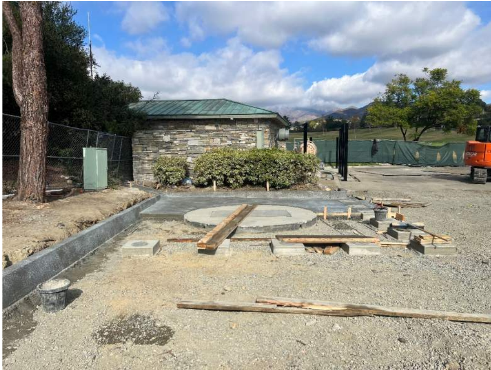
Bypass Wet Well – Concrete Pour for Slab Area
