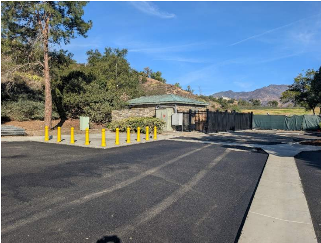
Base Paving Completed; Final Cap, by others (Dove Canyon Golf Club)
