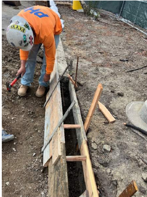
Form Curb & Gutter
