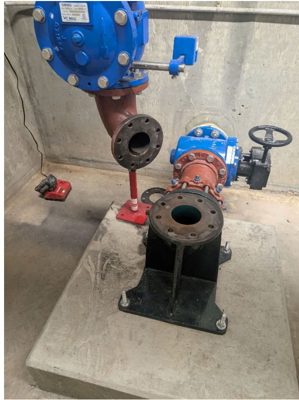
Anchor Bolts Installed
