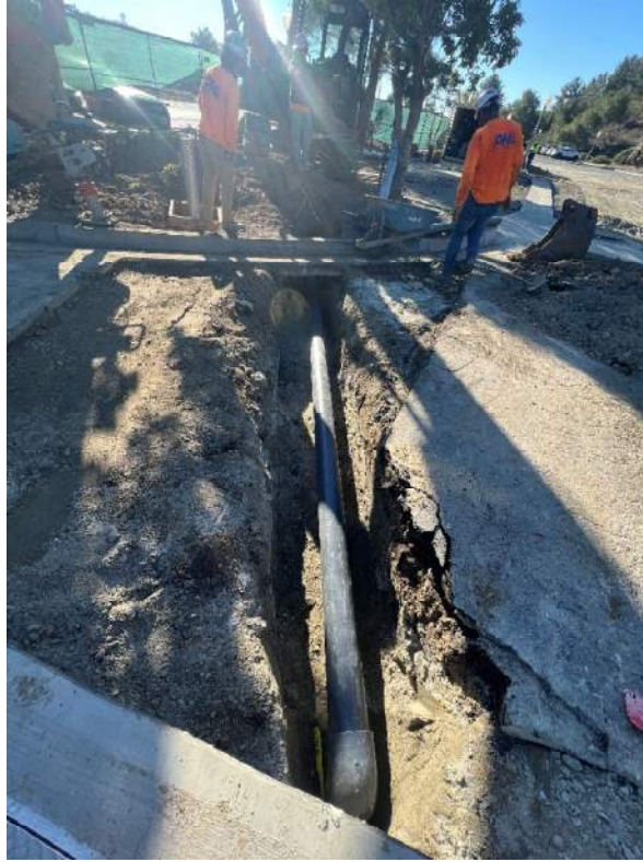
Flow Meter Vault – Install Vent Piping
