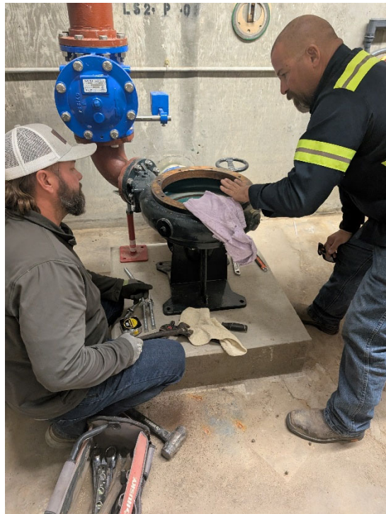
Install Anchor Bolts
