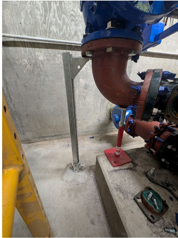
Pipe Stand Installed
