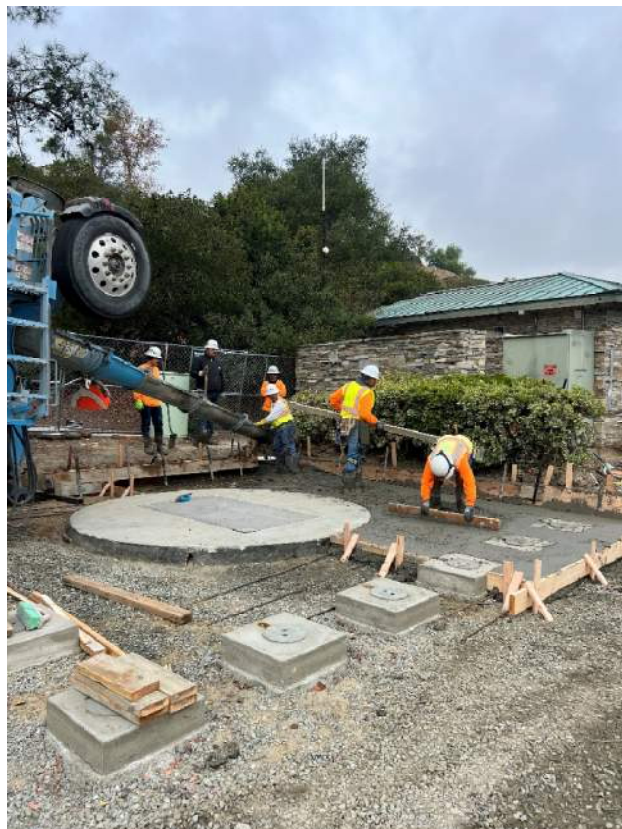
Bypass Wet Well – Concrete Pour for Slab Area
