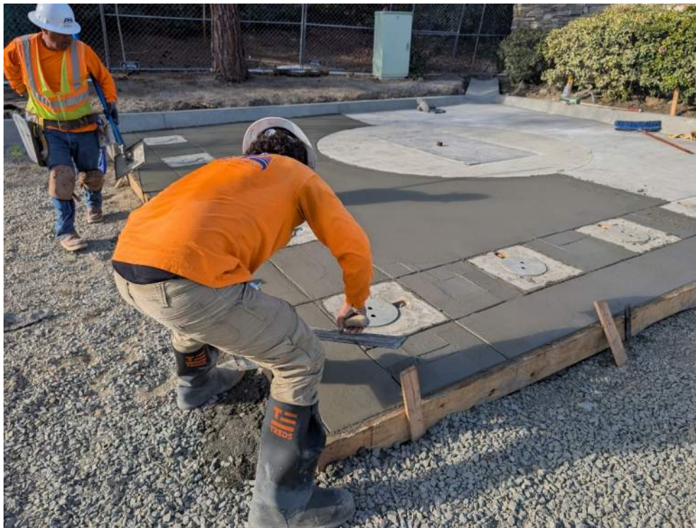
Bypass Wet Well – Concrete Pour for Balance of Slab Area
