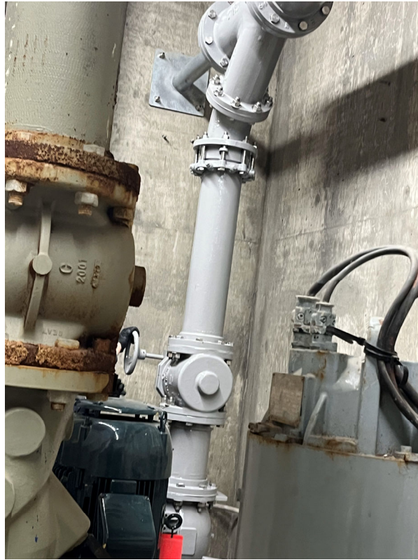
Painting Discharge Manifold Piping
