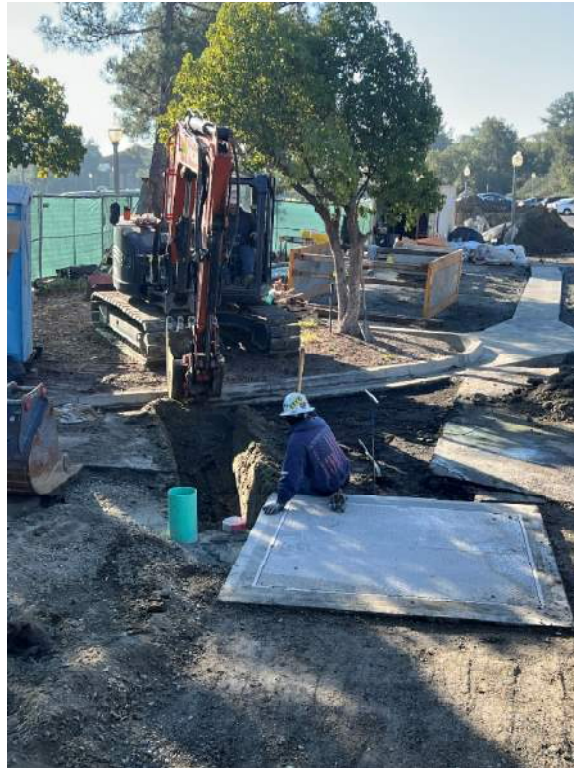
Flow Meter Vault – Excavating to Extend Vent Piping
