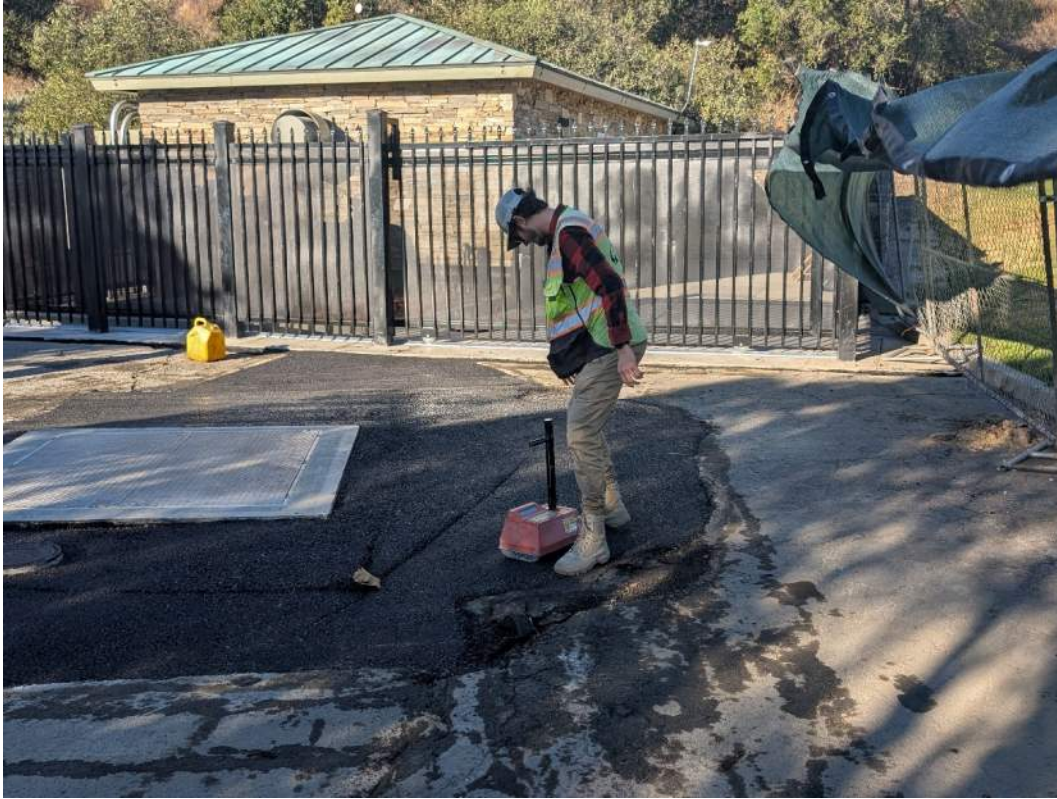
Base Paving Field Compaction Testing
