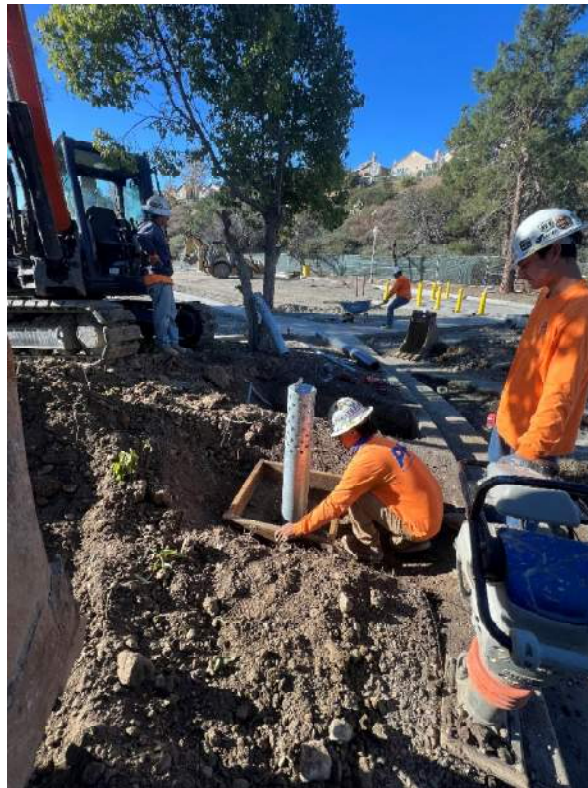
Flow Meter Vault – Complete Install of Vent Piping
