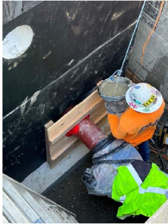
Flow Meter Vault – Wall Repair at Pipe Penetration (“knock-outs”)
