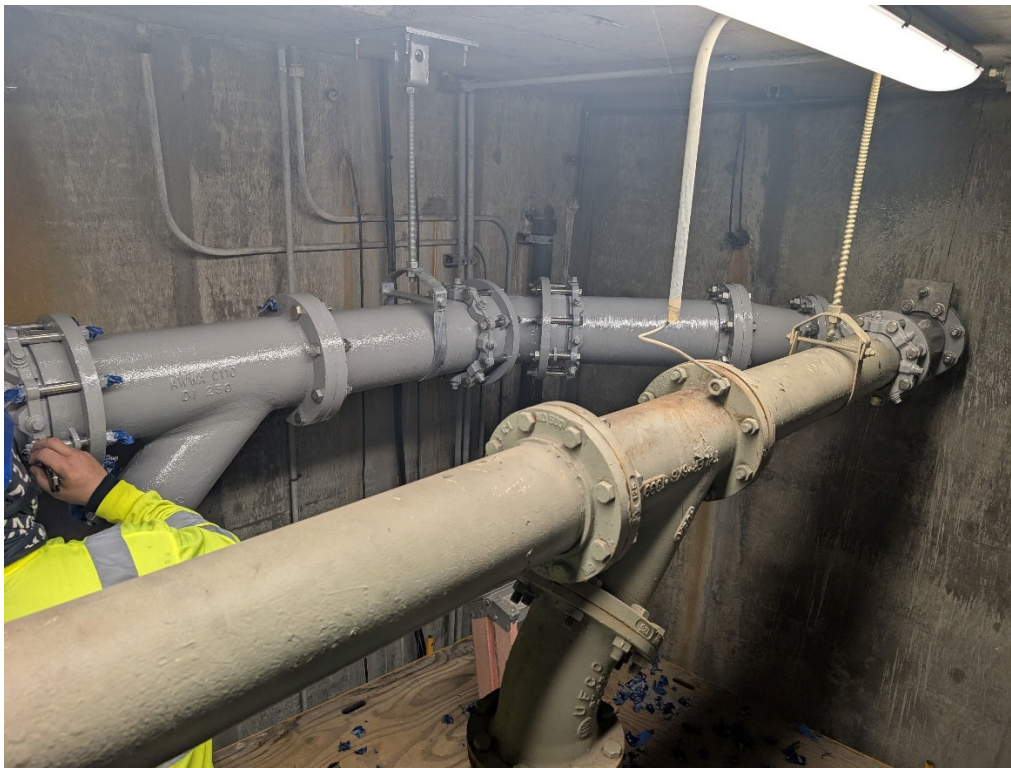
Painting Discharge Manifold Piping
