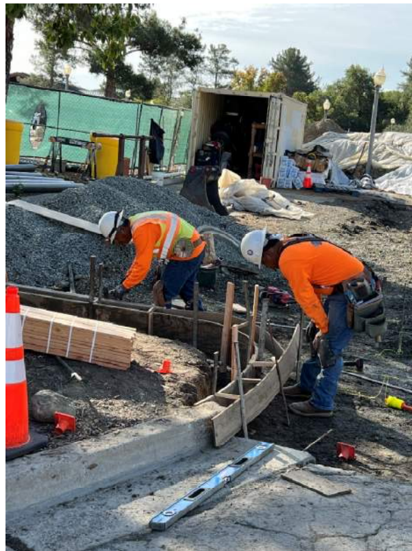
Form Curb & Gutter
