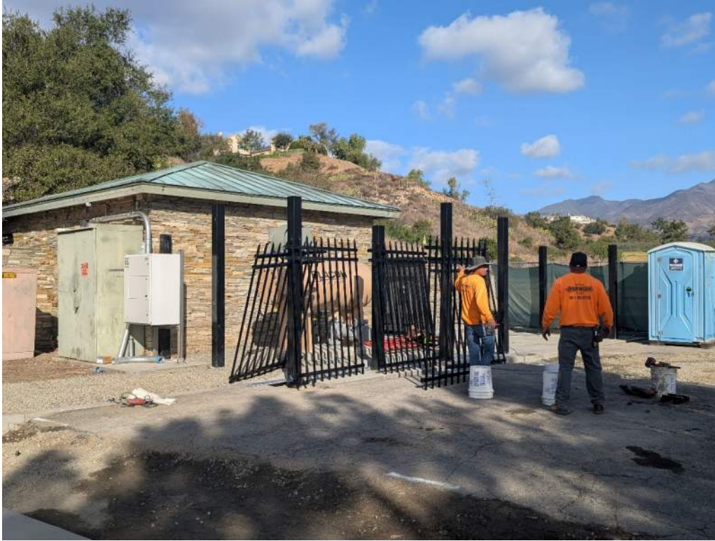
Lift Station – Fence Enclosure & Rolling Gate Installation
