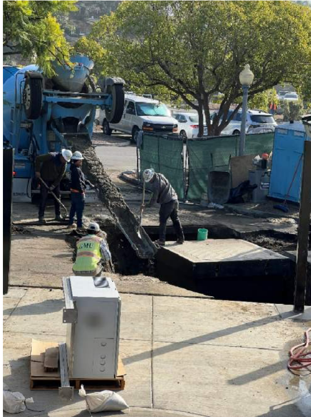
Flow Meter Vault – Slurry Backfill due to Loose Soils
