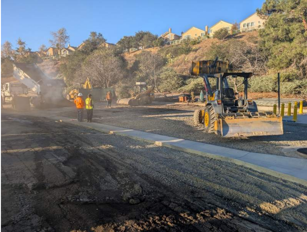
Base Paving Efforts
