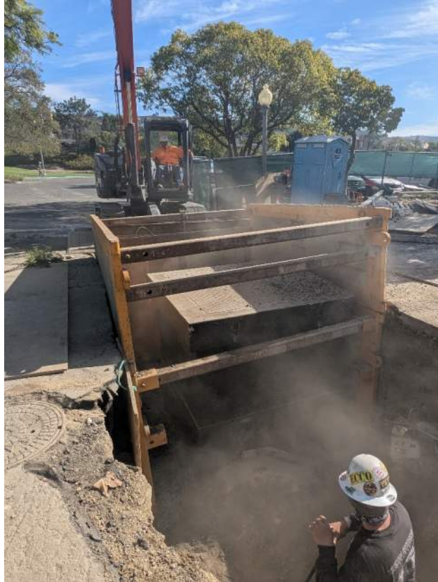
Flow Meter Vault – Shoring Box Removal
