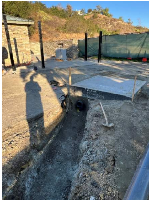
Flow Meter Vault – Install Vent Piping
