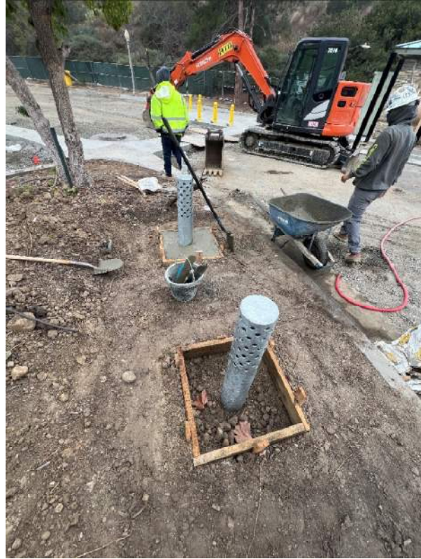
Flow Meter Vault – Finish Vent Piping
