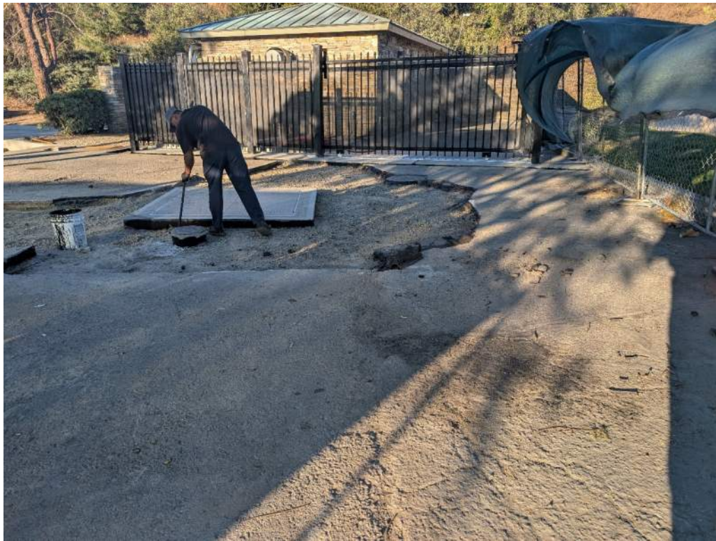
Base Paving Efforts
