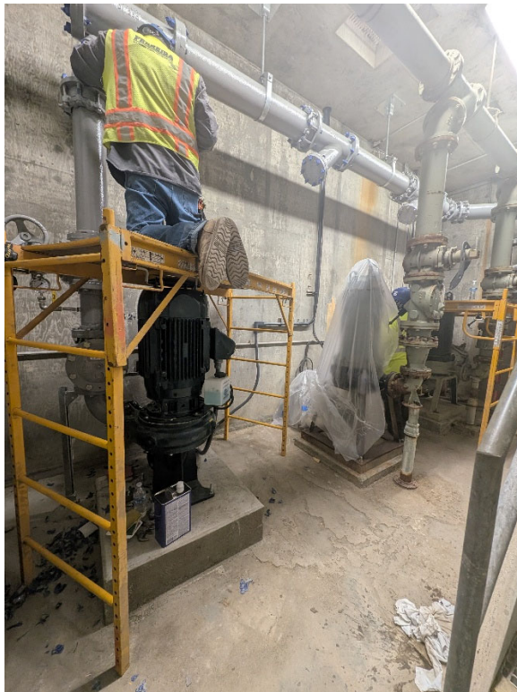
Painting Discharge Manifold Piping
