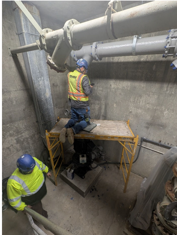
Painting Discharge Manifold Piping
