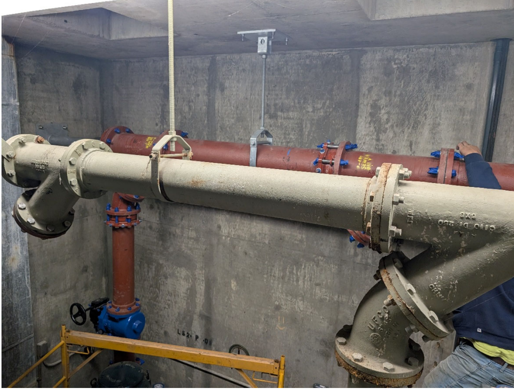
Discharge Manifold Piping Painting Set-Up and Surface Preparation
