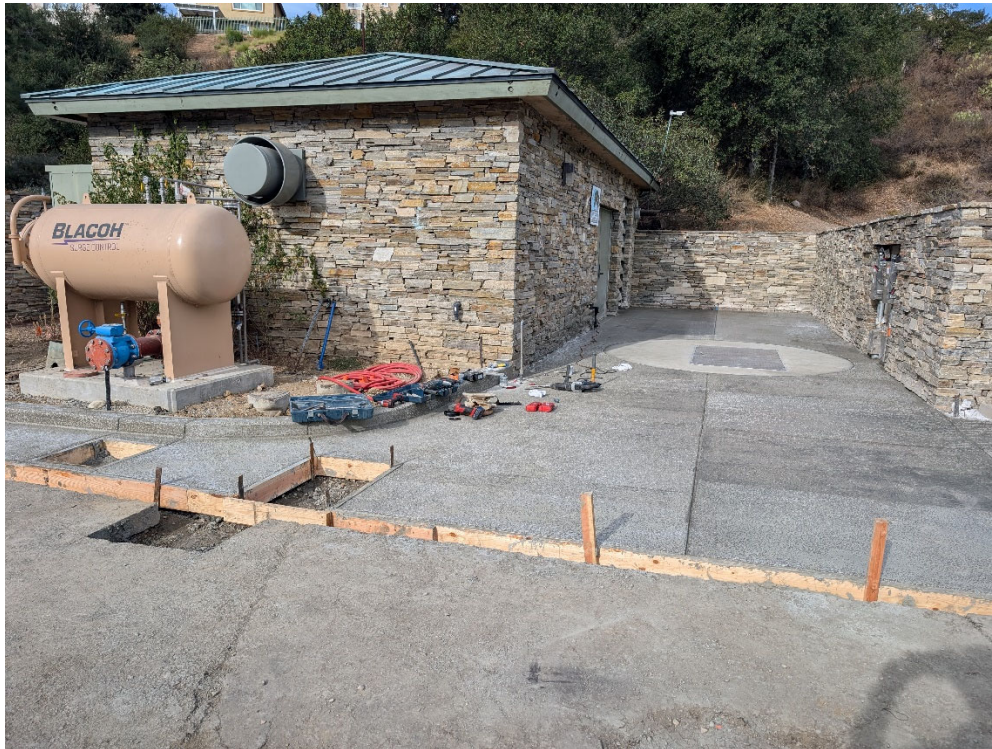
Concrete Curing for Driveway Apron & Roller Gate Track
