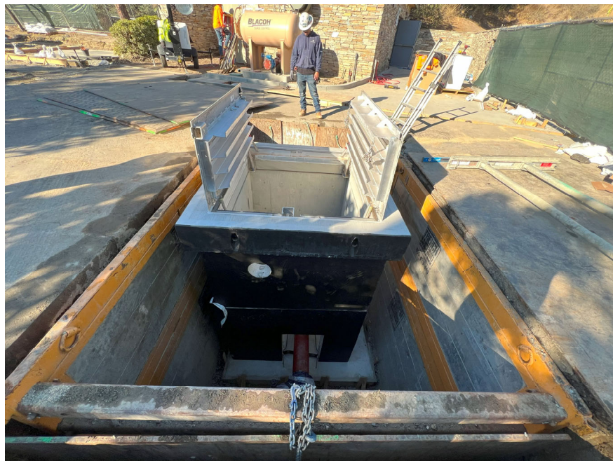
Installation of Flow Meter Vault
