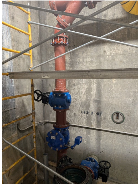
Discharge Manifold Installation and On Pump No. 1
