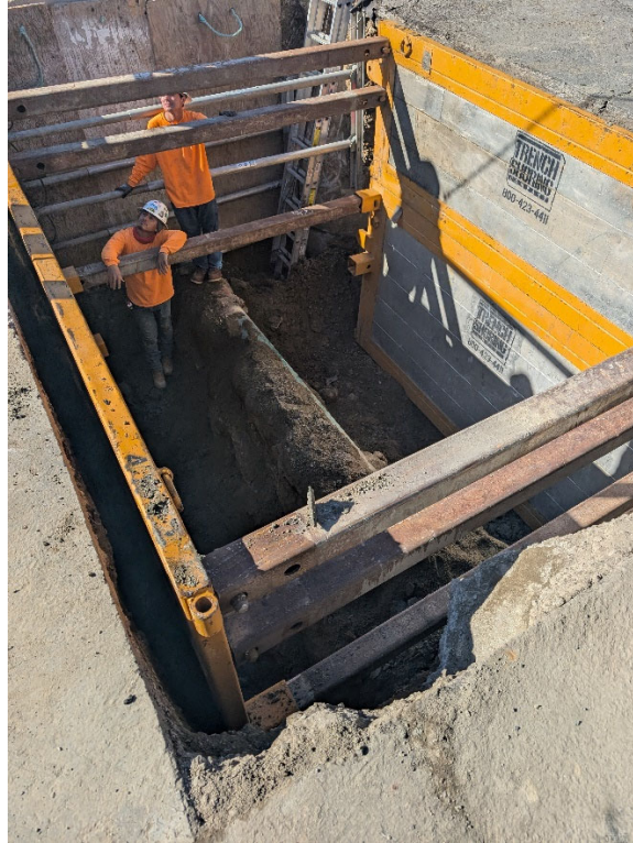
Box Shoring In-Place, and Exposed Existing 8-inch Force Main
