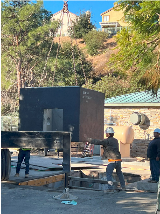
Installation of Flow Meter Vault
