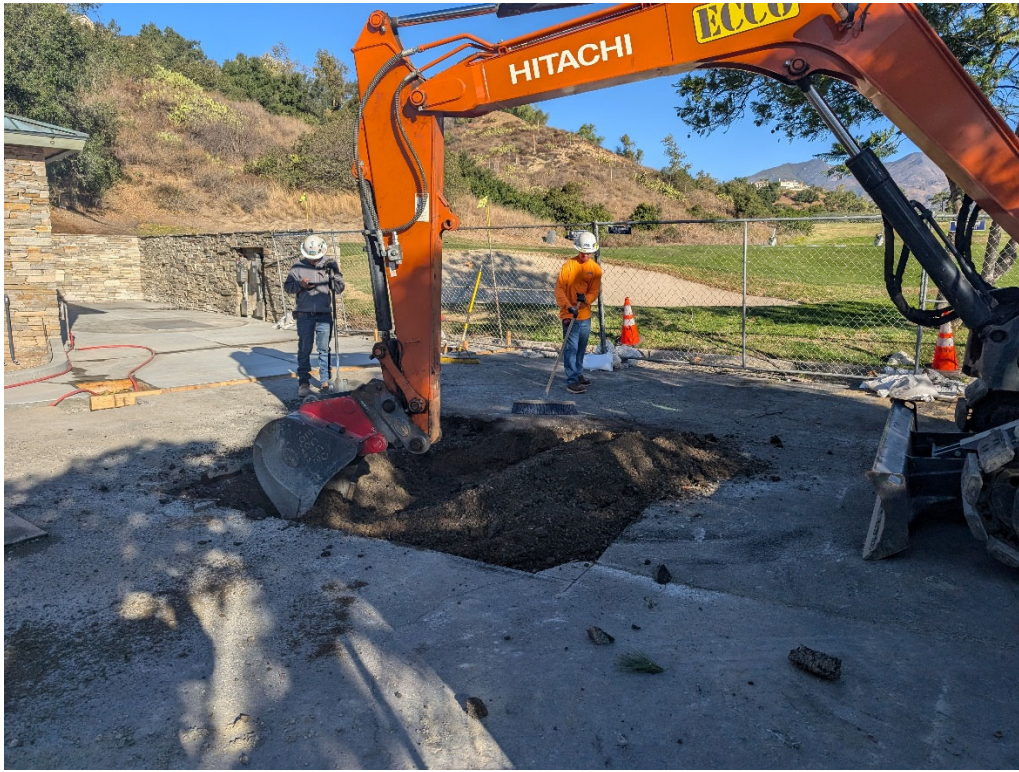
Started Excavation of Flow Meter Vault
