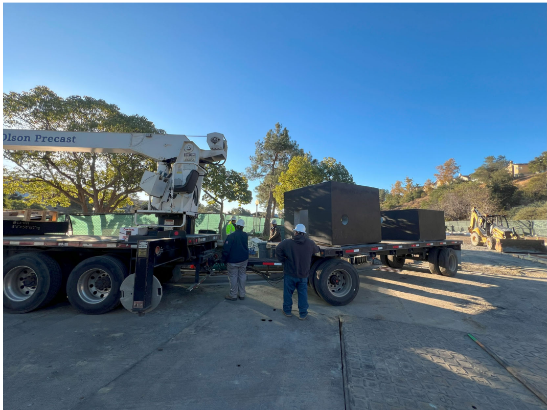
Delivery of Flow Meter Vault
