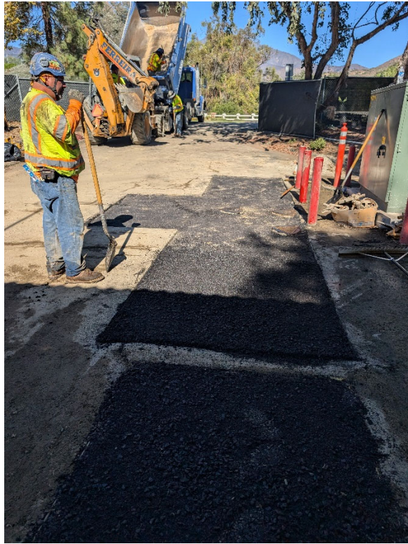
Asphalt Paved Tee Assembly Trench & Air Vac Vault
