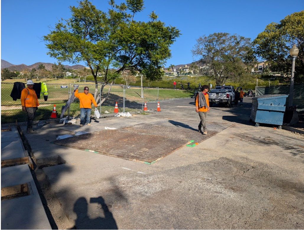
Trench Plates In-Place After Each Work Day
