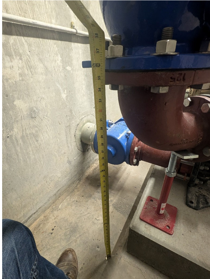
Measurement for New Pipe Support Configuration
