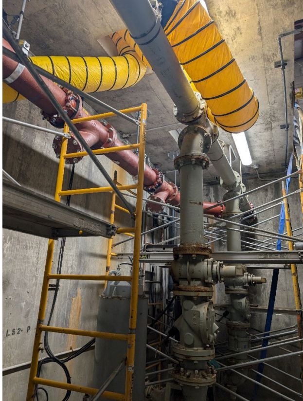
Discharge Manifold Installation
