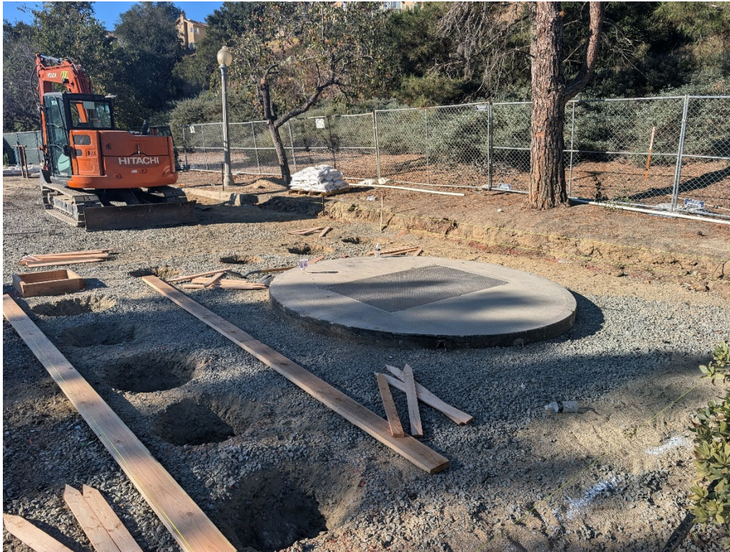
Excavating Bollard Receivers Around Bypass Wet Well
