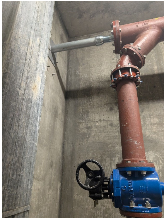
Installed Discharge Manifold Support
