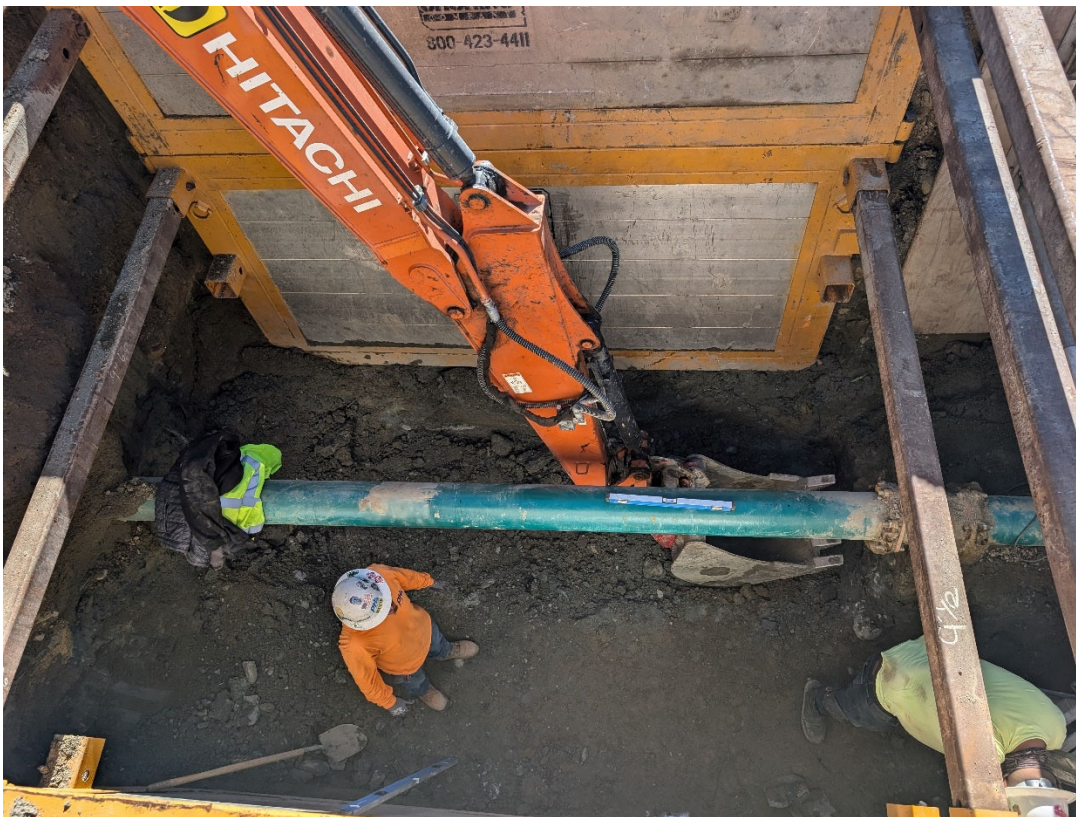
Continue Flow Meter Vault Excavation
