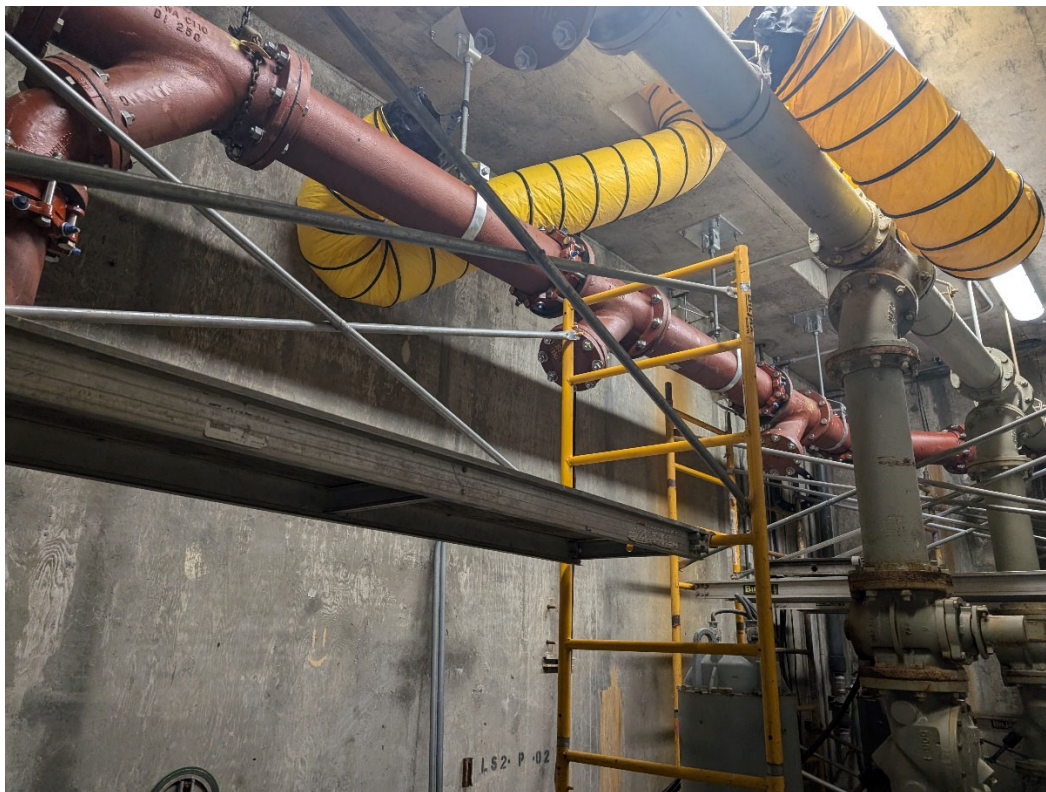
Discharge Manifold Installation
