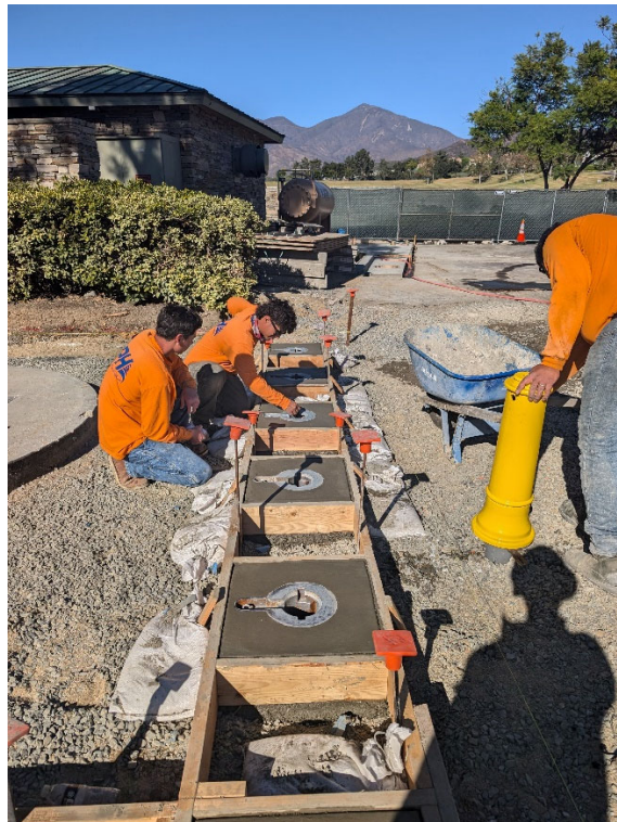
Formed and Poured Concrete for Bollard Receivers Around Bypass Wet Well
