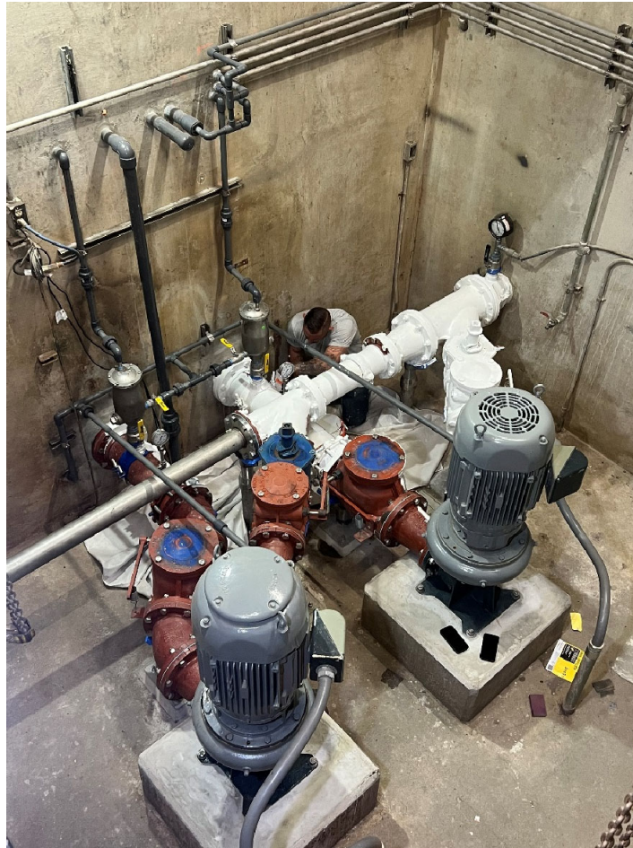
Mechanical Piping Coating with Primer
