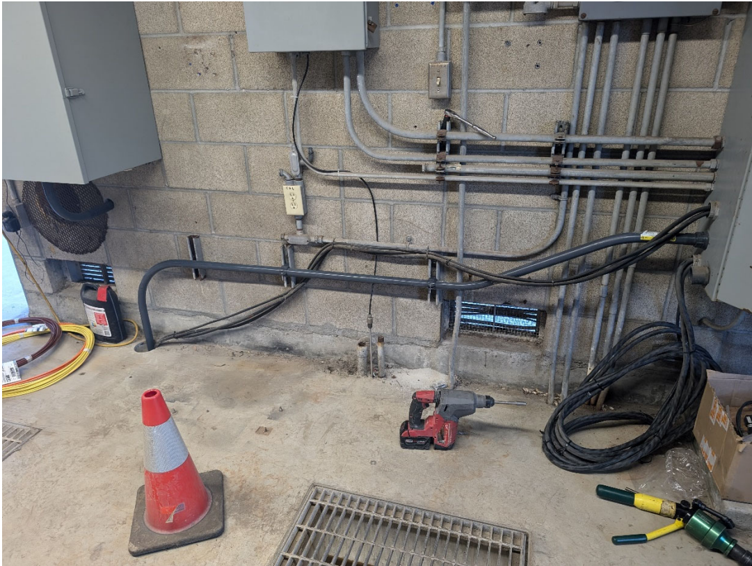
Conduits Installed for Wiring between Pump No. 1 and Motor Control Center
