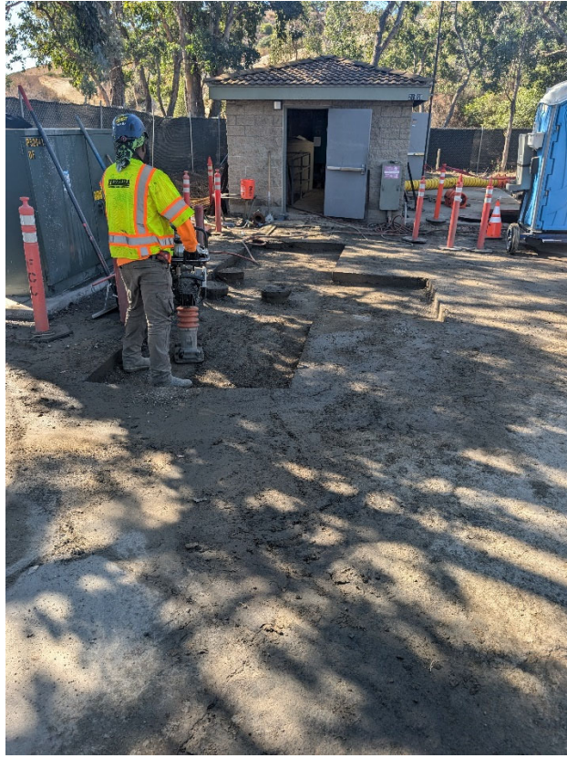
Base Pave Tee Assembly Trench
