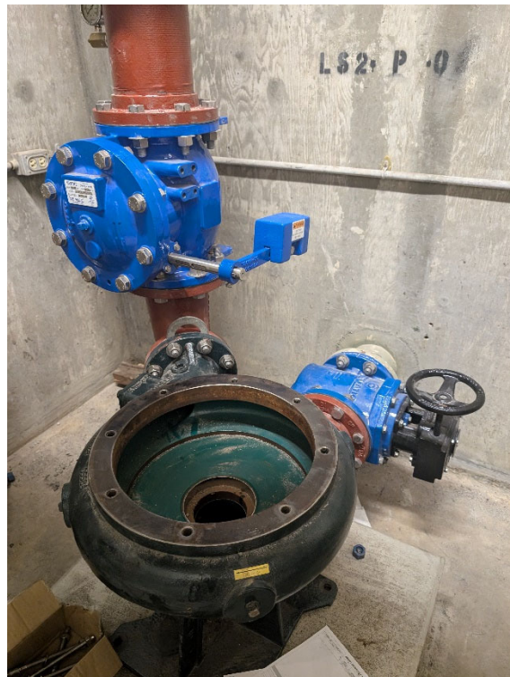
Awaiting Pump No. 1 Install by TCWD Operations
