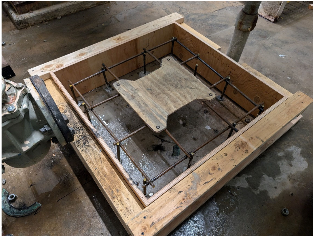
Dry Pit – Form and dowel new Concrete Pad for Pump No. 1.
