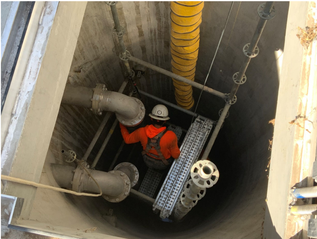
Existing Wet Well – TECHNO Coatings remobilized and started lining application; Scaffolding being installed.
