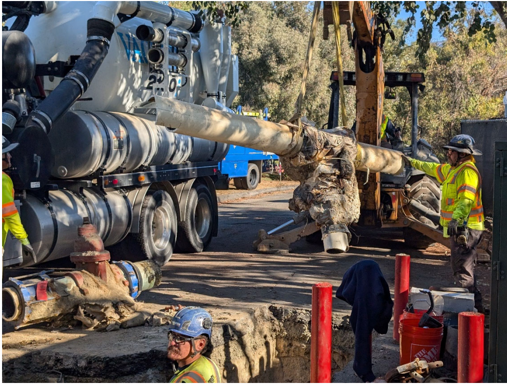
Cut-In Tee & Plug Valves Assembly – Removal of Existing Tee.
