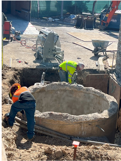
Existing Wet Well – Penhall getting ready to clean-cut top of Wet Well.
