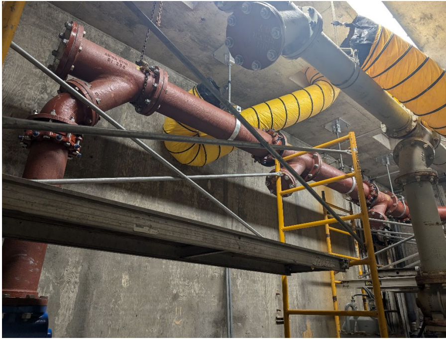
Dry Pit – Discharge Manifold Being Installed
