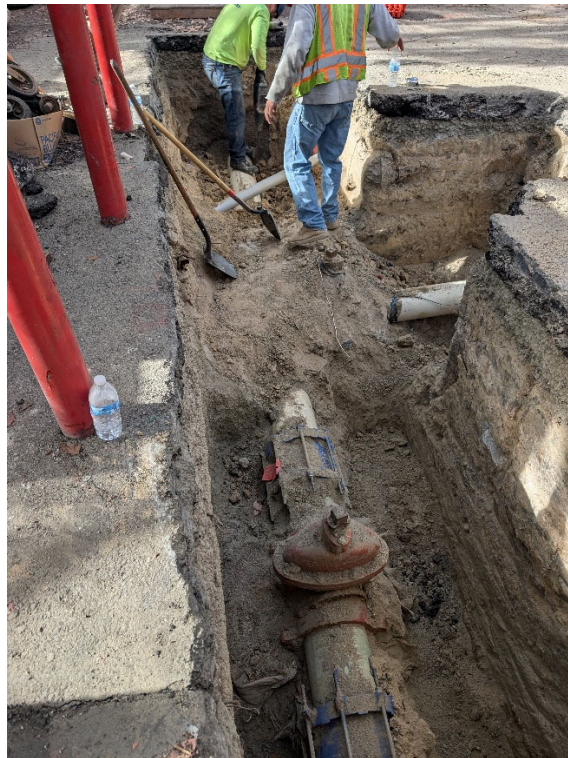
Cut-In Tee & Plug Valves Assembly – Started excavation and exposed existing tee connection; notice 3-inch SCE Conduit crossing pipeline and protected-in-place.
