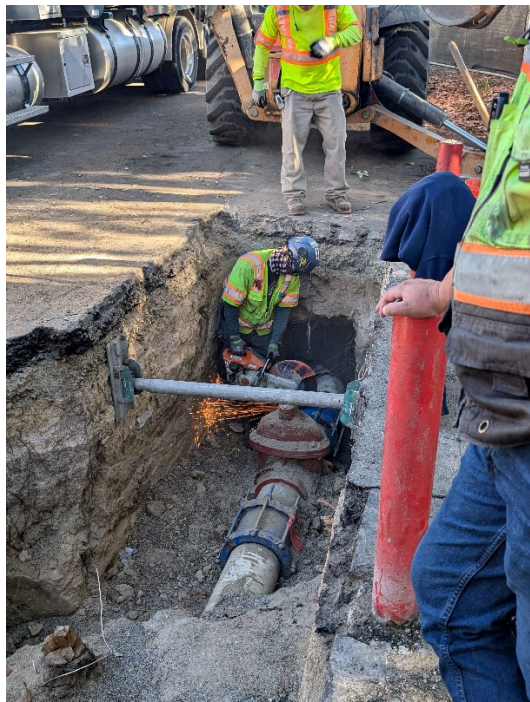
2 nd Shut Down – Cut-In Windows/Ports for Vector Truck Snorkel Access.
