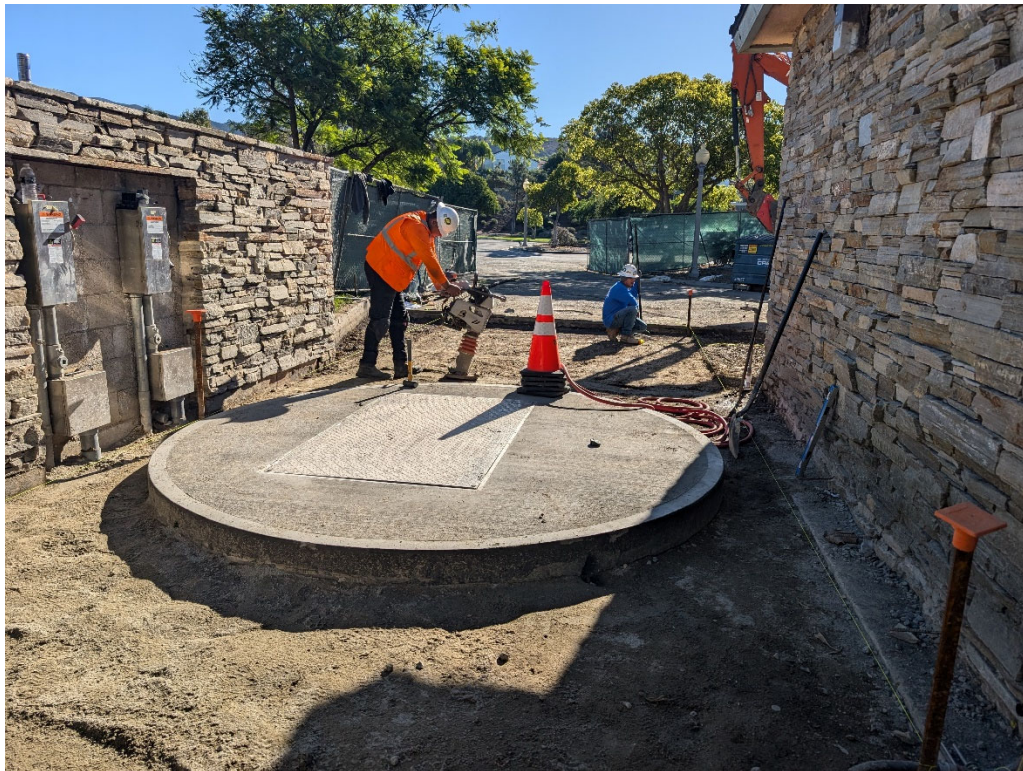
Existing Wet Well – Grading and compacting areas to be received with concrete slab improvements.
