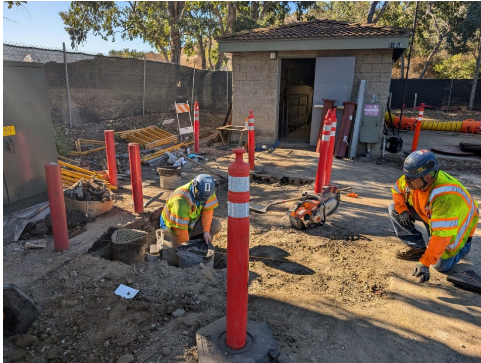
Cut-In Tee & Plug Valves Assembly – Installing Valve Boxes & Covers
