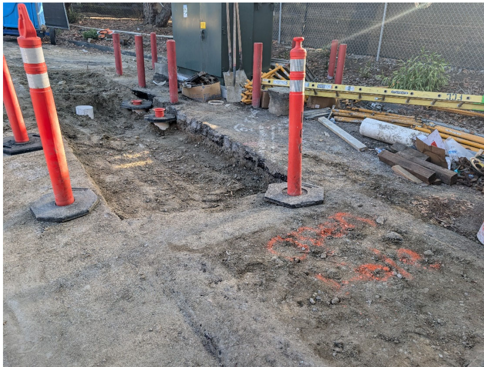
Cut-In Tee & Plug Valves Assembly – Backfilled Excavation; Field Compaction Testing by GMU.
