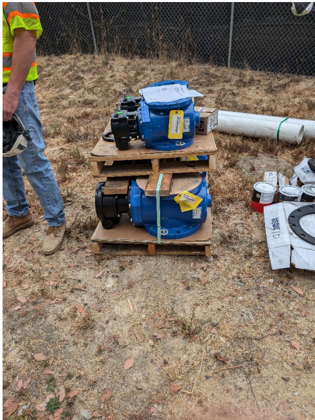
Heritage Lift Station – Materials being delivered by Western Waterworks.
