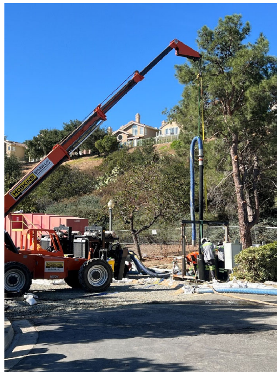
Golf Club Lift Station – Decommissioning of Temporary Bypass System
