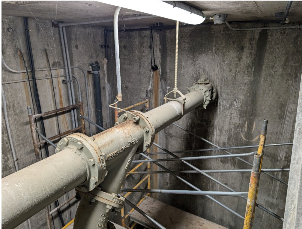
Dry Pit – Scaffolding and preparation of 6x6 Wye at Discharge Header.
