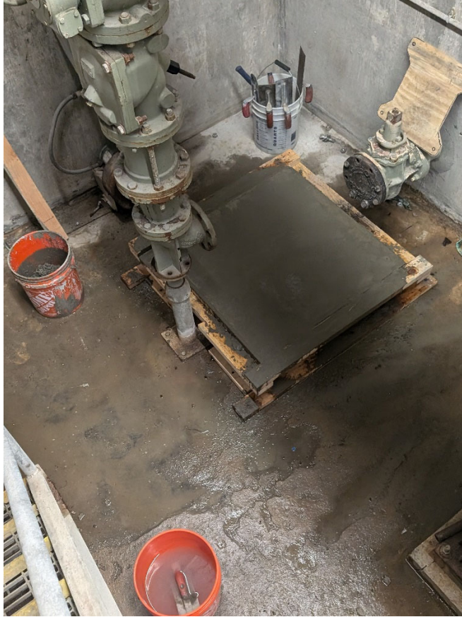
Dry Pit – Poured Concrete Pad for Pump No. 1.
