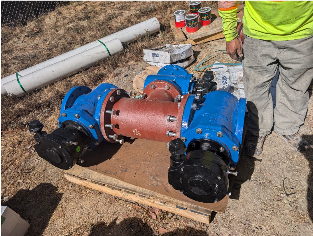
Cut-In Tee & Plug Valves Assembly – Started assembling and staging.
