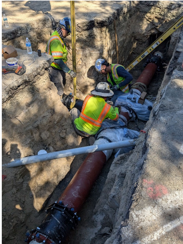
Cut-In Tee & Plug Valves Assembly – New Tee Assembly Installed; Wrapped Valves
