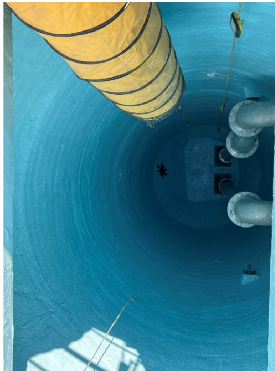
Existing Wet Well – Lining application completed.
