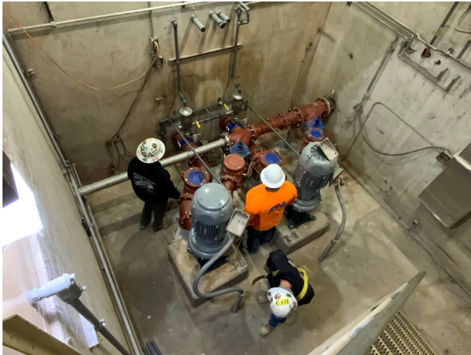
Existing Dry Well – Pump Motors replaced; electrical connections and terminations performed by Hydrotech Electric.
