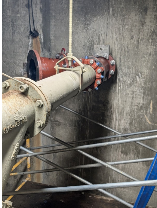
Dry Pit – Installed 6x6 Wye for new Discharge Header Pipe
