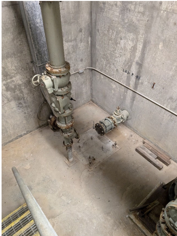
Dry Pit – Removal of Concrete Pad
