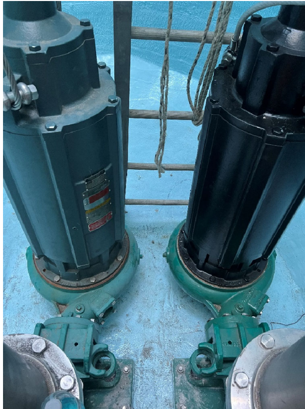
Existing Wet Well – Placement of Submersible Pumps; Electrical connections being made by Hydrotech Electric.
