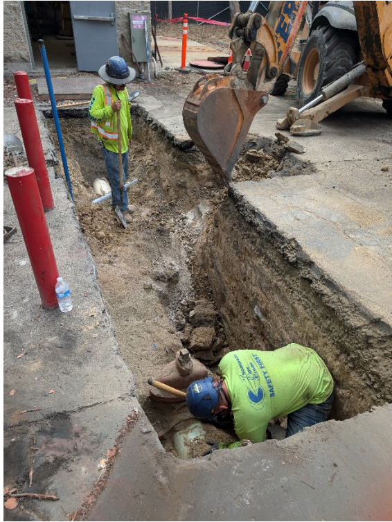
Cut-In Tee & Plug Valves Assembly – Started excavation and expose existing tee connection.
