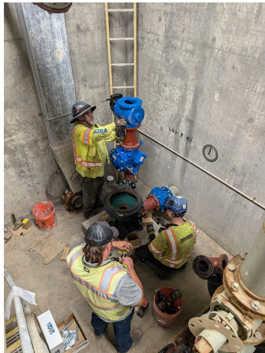
Dry Pit – Assembling Pump, Piping, and Valves
