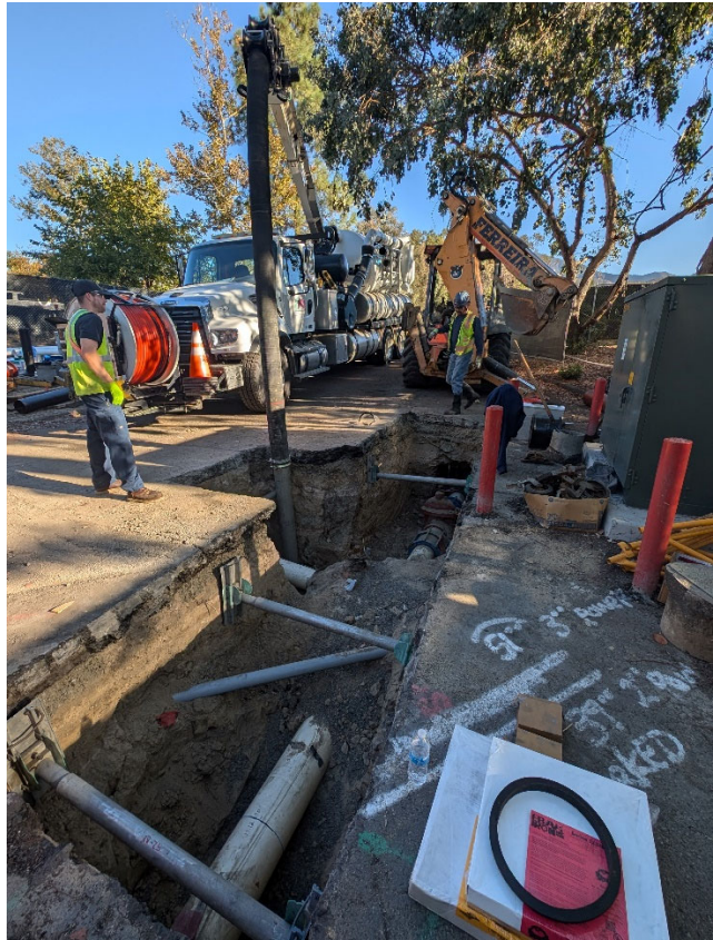
2 nd Shut Down – Vector Truck mobilized near Excavated Tee Assembly
