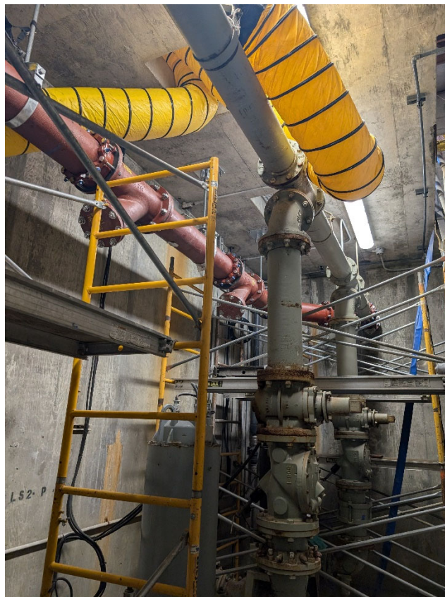
Dry Pit – Discharge Manifold Being Installed
