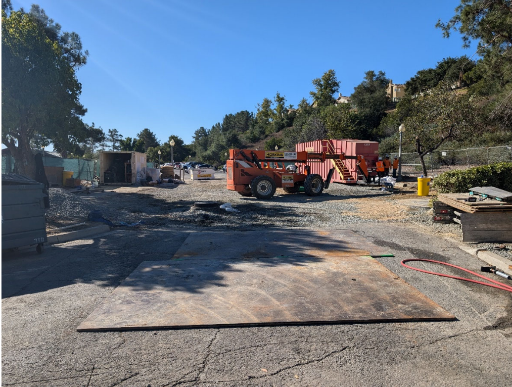
Golf Club Lift Station – Decommissioning of Temporary Bypass System.
