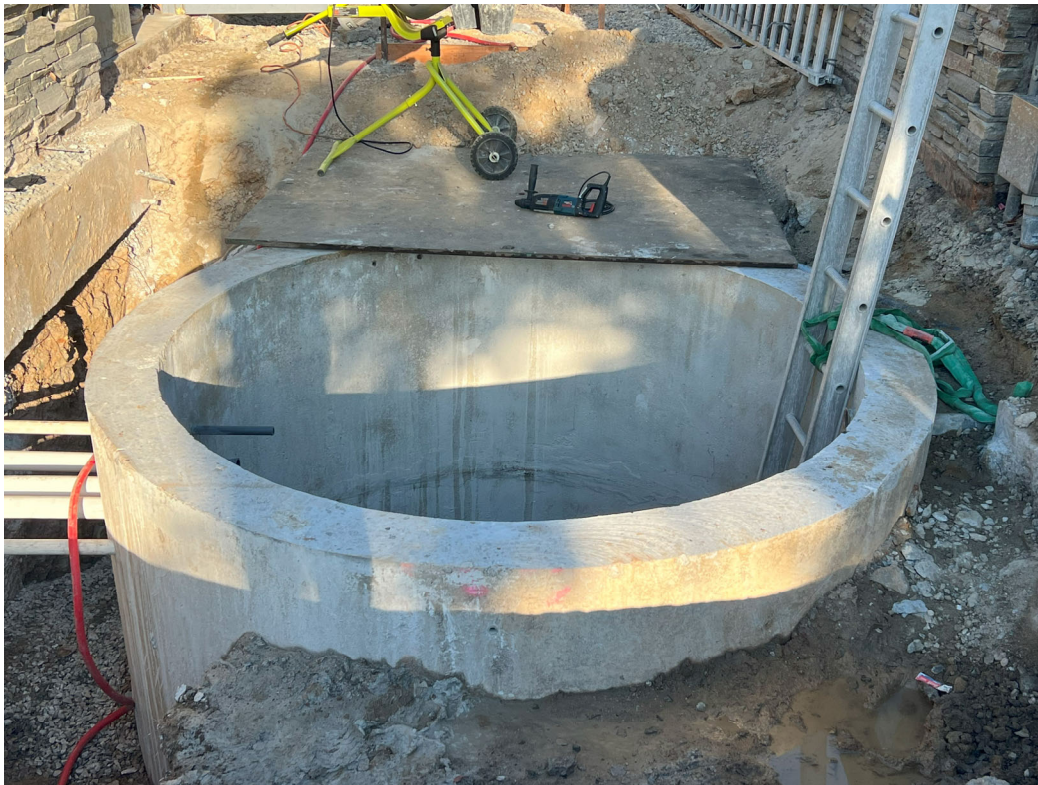
Existing Wet Well – result of a clean-cut Wet Well prior to Pre-Cast Slab/Hatch placement.
