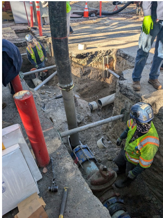
2 nd Shut Down – Cut-In Windows/Ports for Vactor Truck Snorkel Access.
