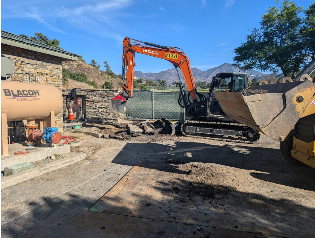
Existing Wet Well – Asphalt removals for concrete slab placement.
