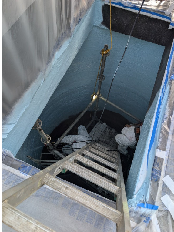
Existing Wet Well – TECHNO continuing to apply lining application.
