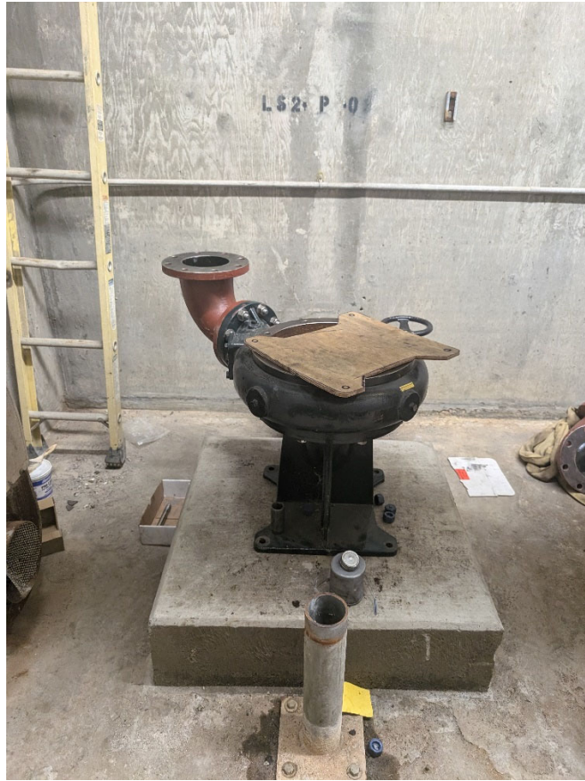
Dry Pit – Setting Pump
