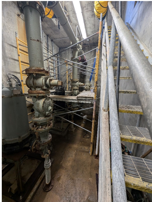
Dry Pit – Scaffolding Installed and Prepared
