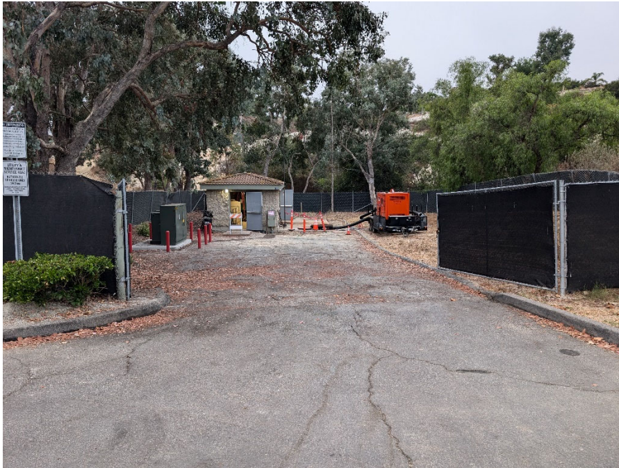
Heritage Lift Station – Mobilizing onto project site.
