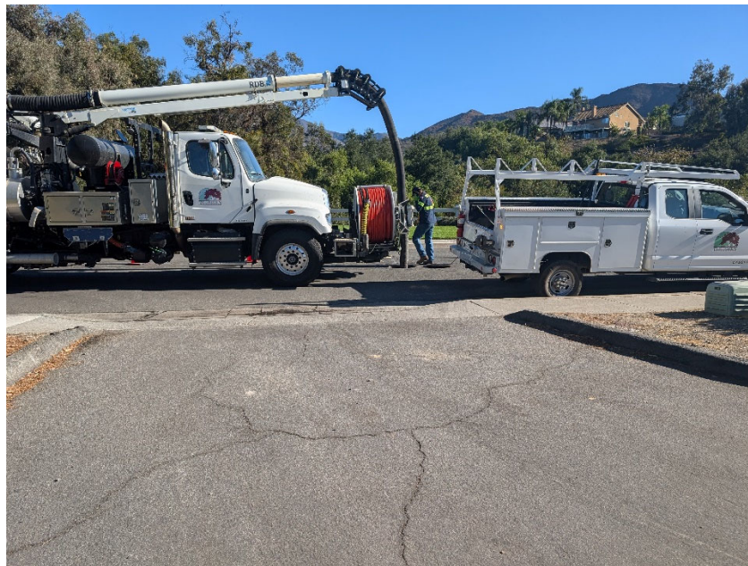
1 st Shut Down – Vector Truck on site.
