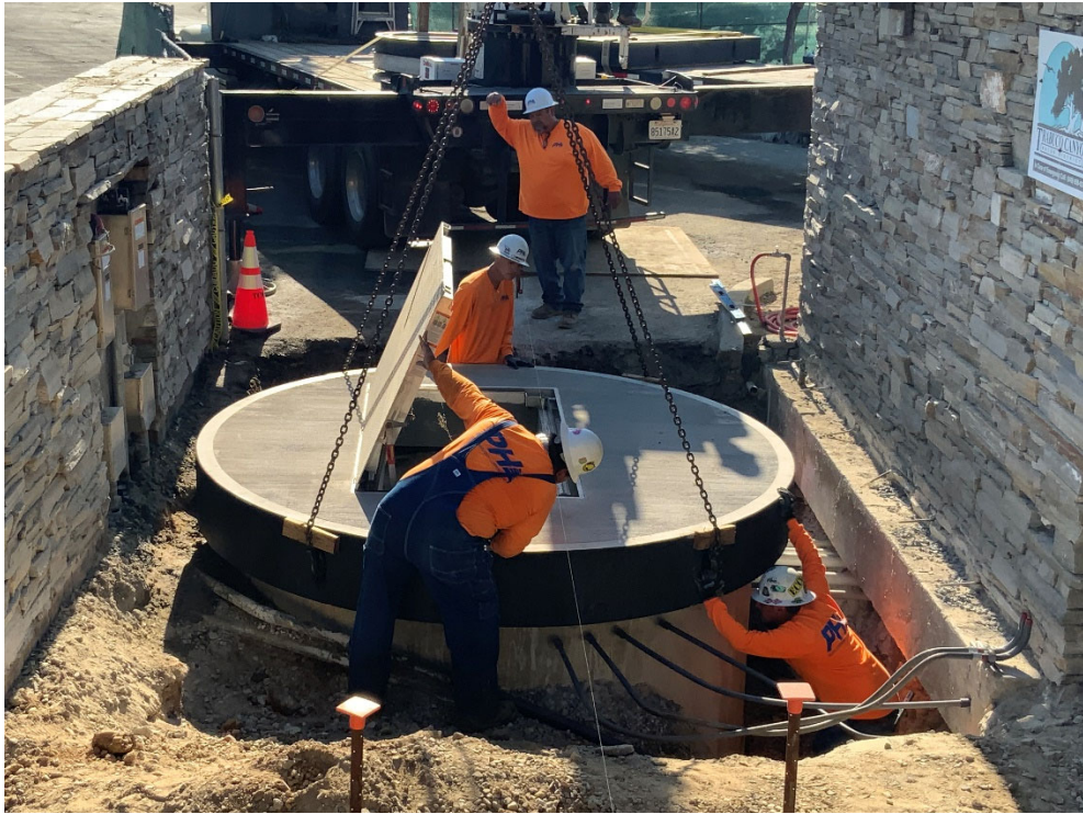
Existing Wet Well – Placement of Pre-Cast, Lid & Hatch.
