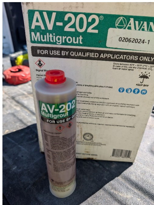
Existing Wet Well – where any leakage from the interior, concrete walls were observed, TECHNO injected a Multigrout application.
