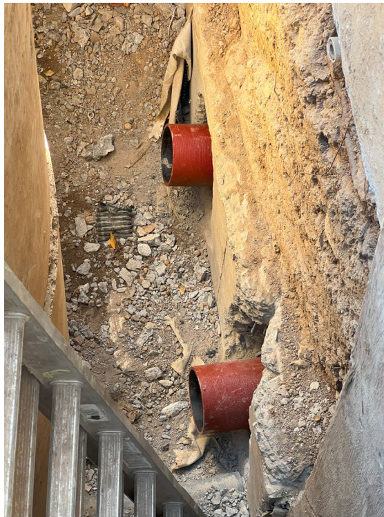
Dry Well – Ductile iron pipe installed through penetrations of Dry Well.
