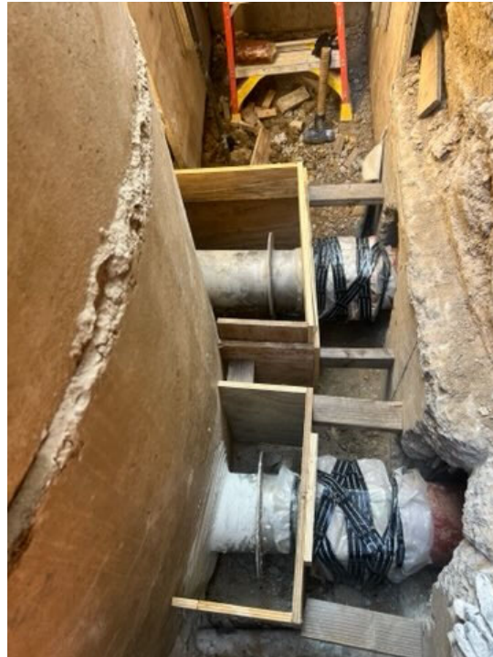
Existing Wet Well & Dry Well – Form-and-pour concrete collars.
