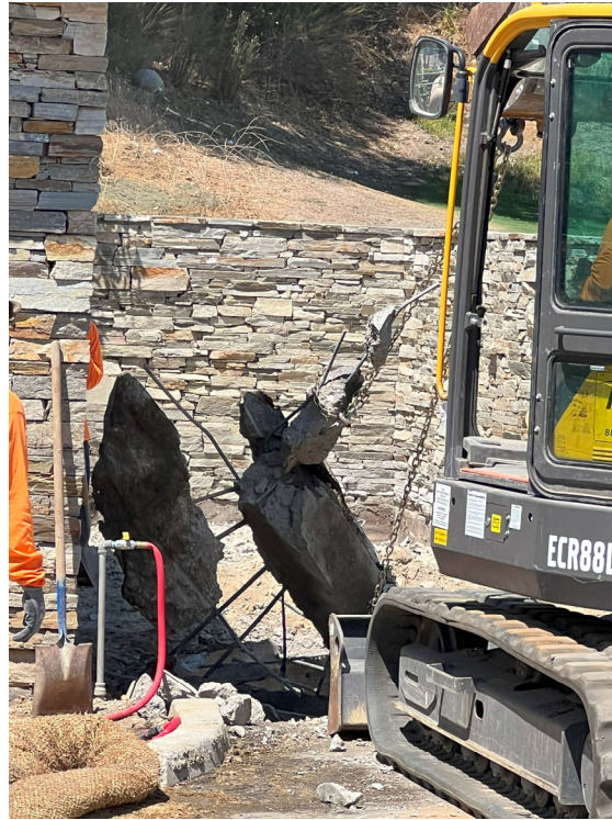
Existing Wet Well – Hardscape removals.
