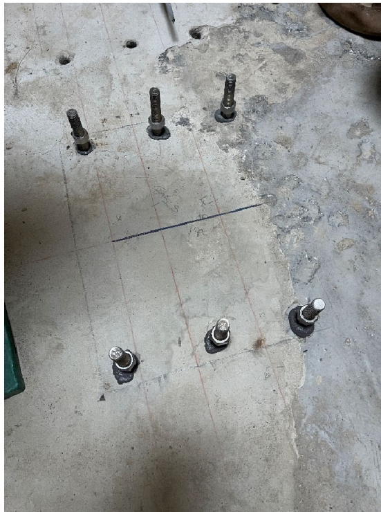
Existing Wet Well – Pump Base template and bolt extensions set.
