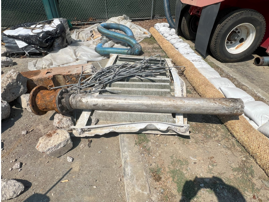
Existing Wet Well – Pipe removals.
