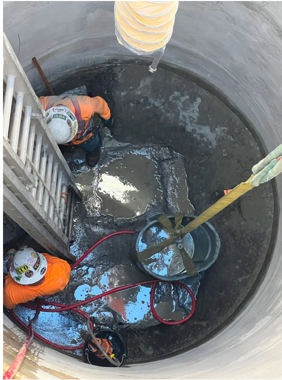
Existing Wet Well – Removal of Concrete Chamfer Slope.
