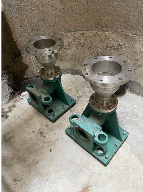
Existing Wet Well – Pump Bases set.
