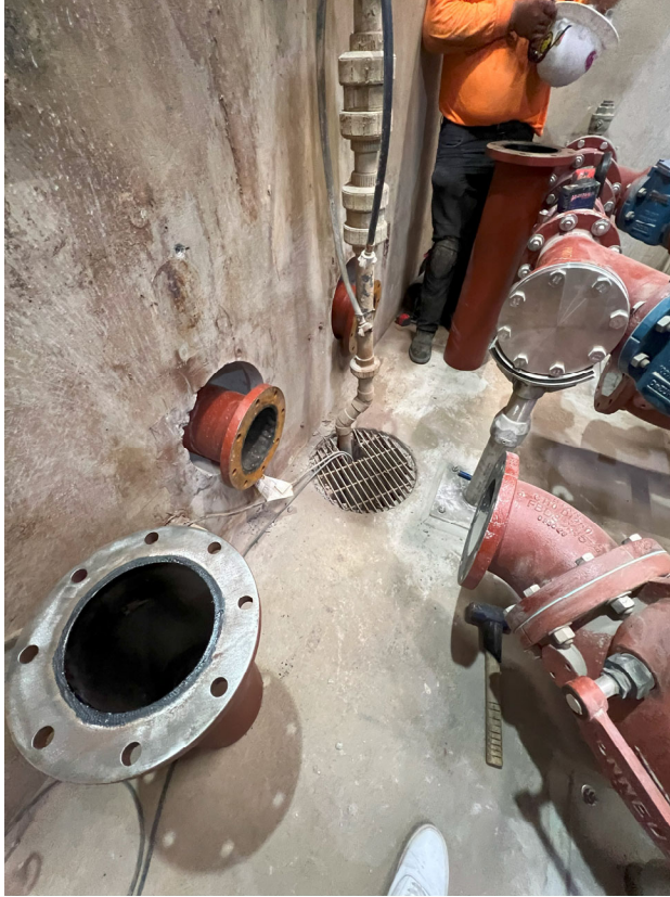
Dry Well – PHC installed ductile iron pipe through Dry Well.
