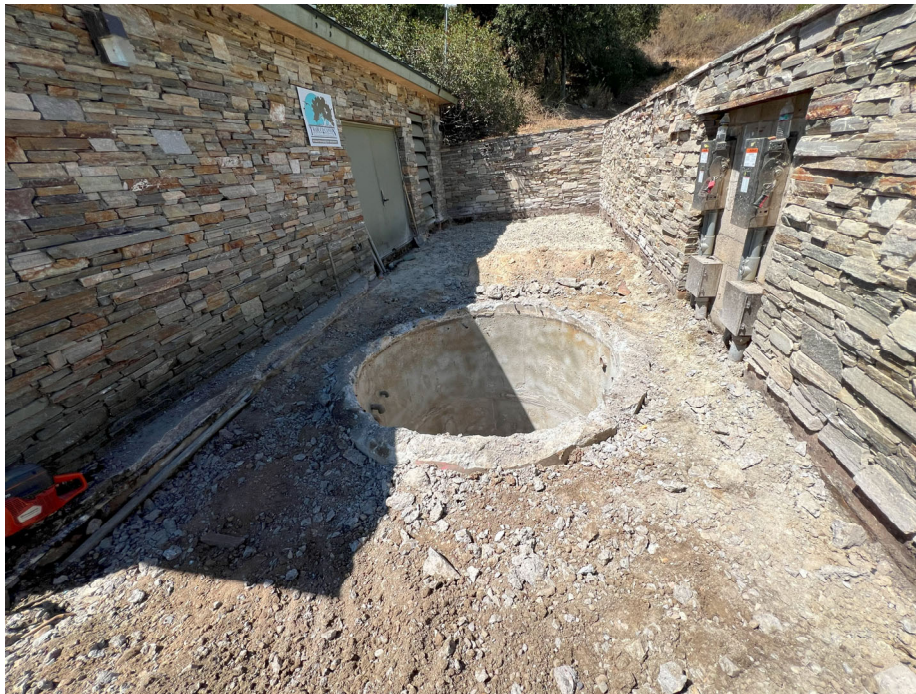
Existing Wet Well – Removals of hardscape completed.
