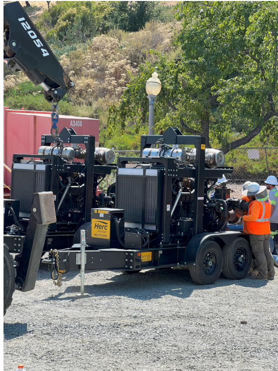
Temporary Bypass System – PHC and HERC continued installation of Bypass System.
