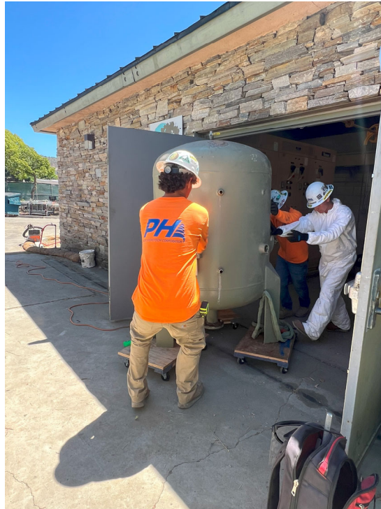
Existing Dry Well – pre-existing Surge Tank being removed.
