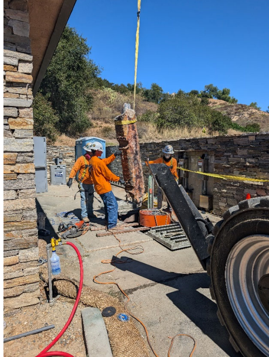
Existing Wet Well – removals being performed.
