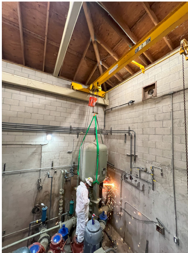
Existing Dry Well – removals being performed, pre-existing Surge Tank being removed.
