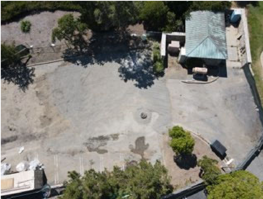
Temporary Demobilization, Project Site – site secured.
