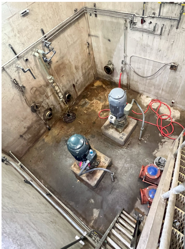
Existing Dry Well – removals being performed.
