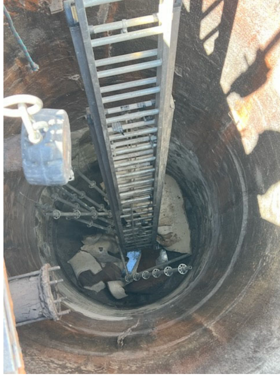
Existing Wet Well – Techno Coatings placing scaffolding.
