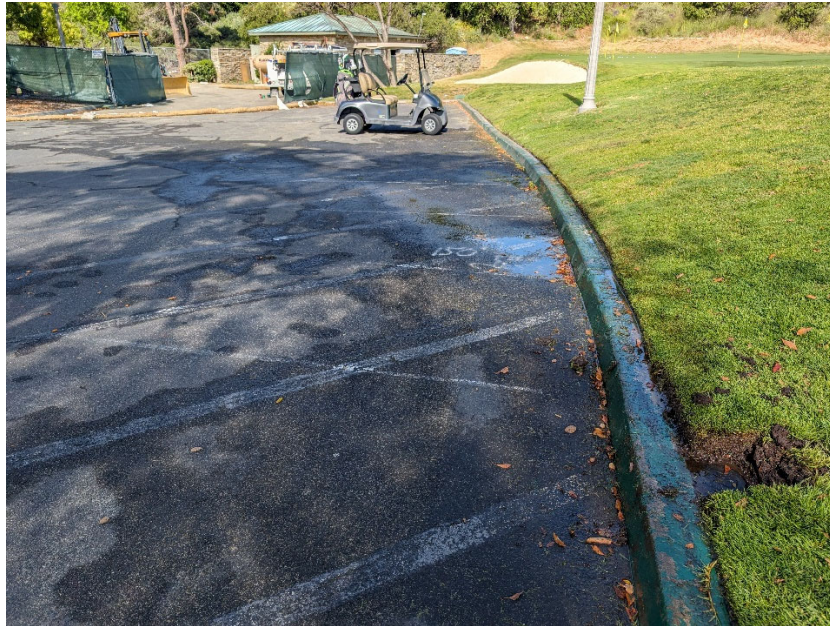
Temporary Demobilization, Project Site – Golf Club surface drainage runoff from irrigation.
