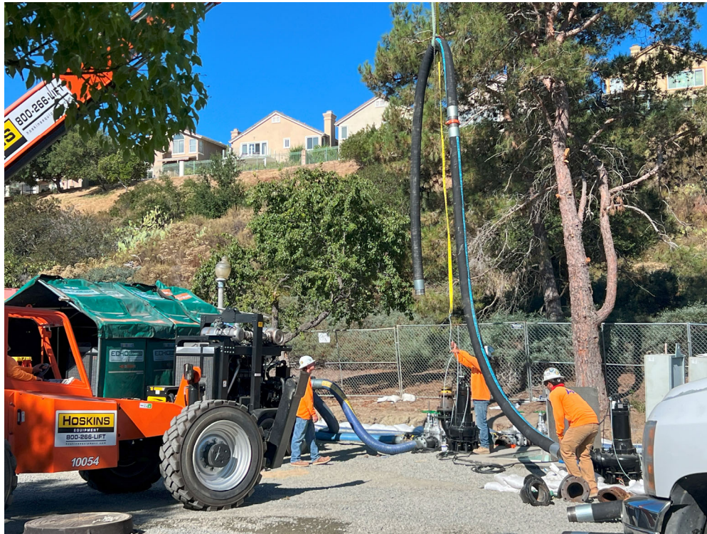
Temporary Bypass System – PHC and HERC continued installation of Bypass System.
