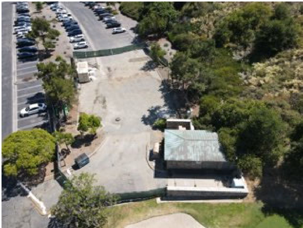
Temporary Demobilization, Project Site – site secured.
