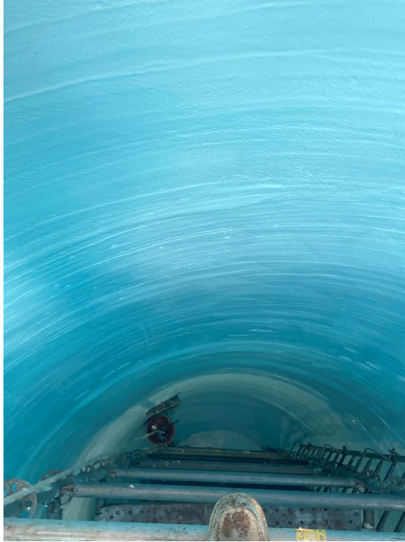
Bypass Wet Well – interior with epoxy lining application.
