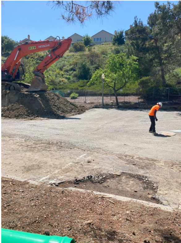
Continued placement of Aggregate Base Material
