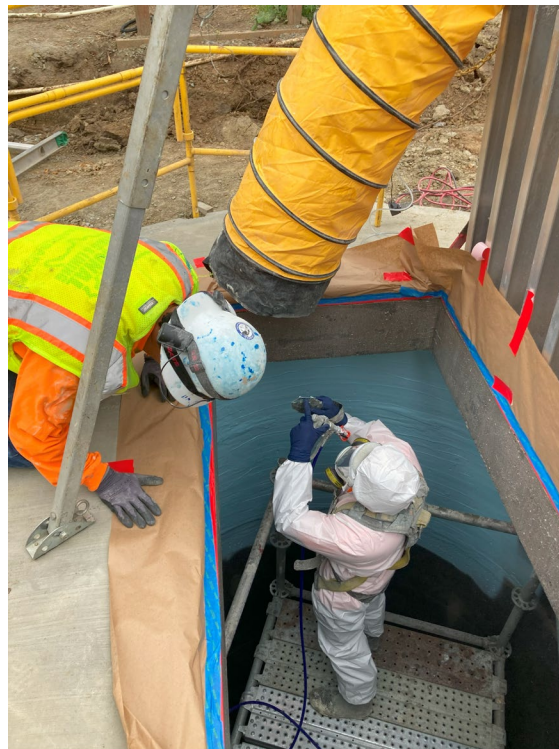
Bypass Wet Well – Techno Coatings applying Raven Epoxy Lining system.
