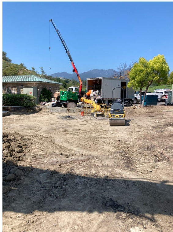
Subgrade being graded and prepared for aggregate base material placement.
