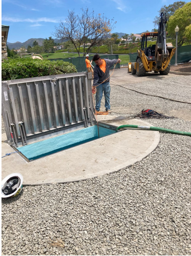
Securing substructures in preparation for temporary demobilization.
