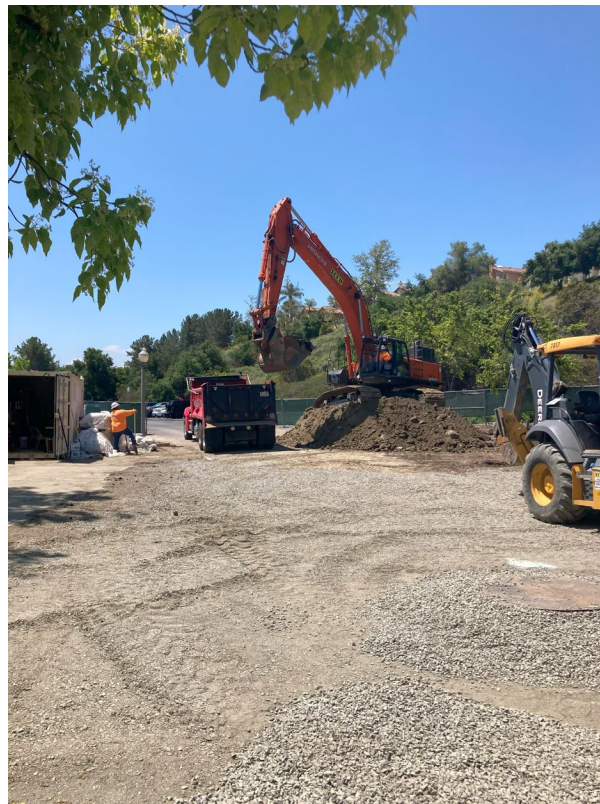
Hauled-off surplus, excavated materials.
