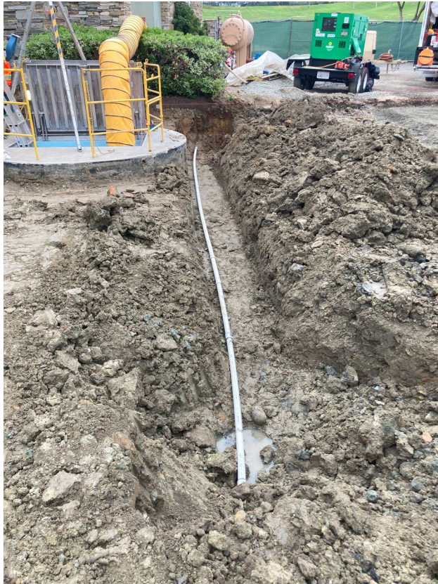
Unmarked Domestic Water Line – PHC performing repairs and realignment.
