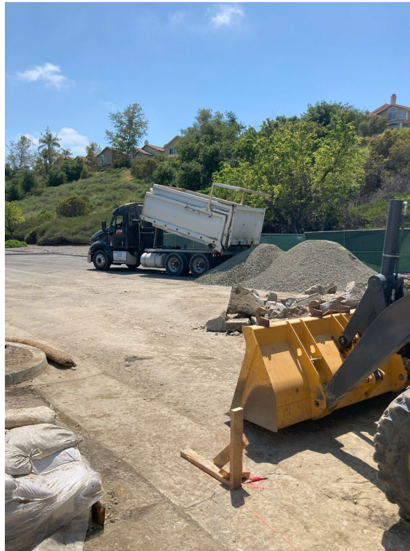
Aggregate Base Material being delivered to project site.
