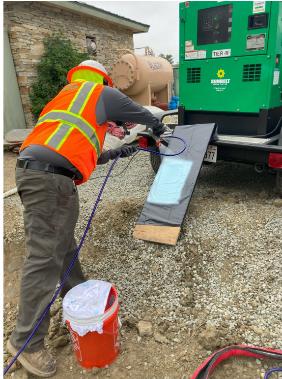
Bypass Wet Well – mock-up of Raven Epoxy Lining system.
