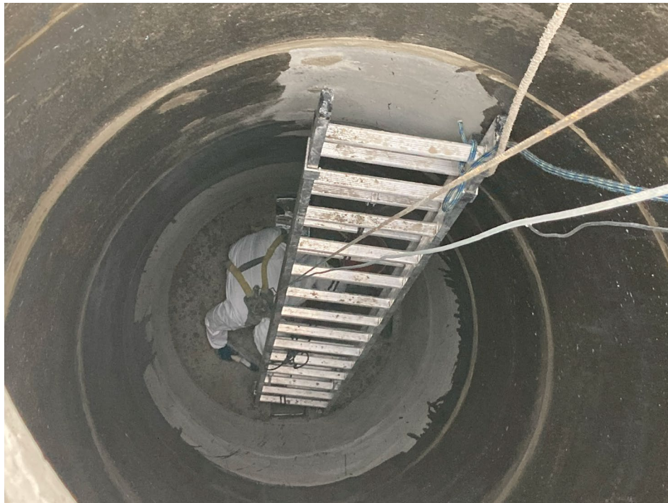
Diversion Manhole – Techno Coatings applying primer within the interior walls.
