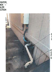
SEWER CLEANOUT PHOTO 2 NTS
