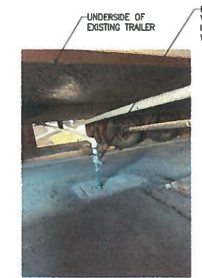
METER BOX CONNECTION PHOTO 1 NTS
