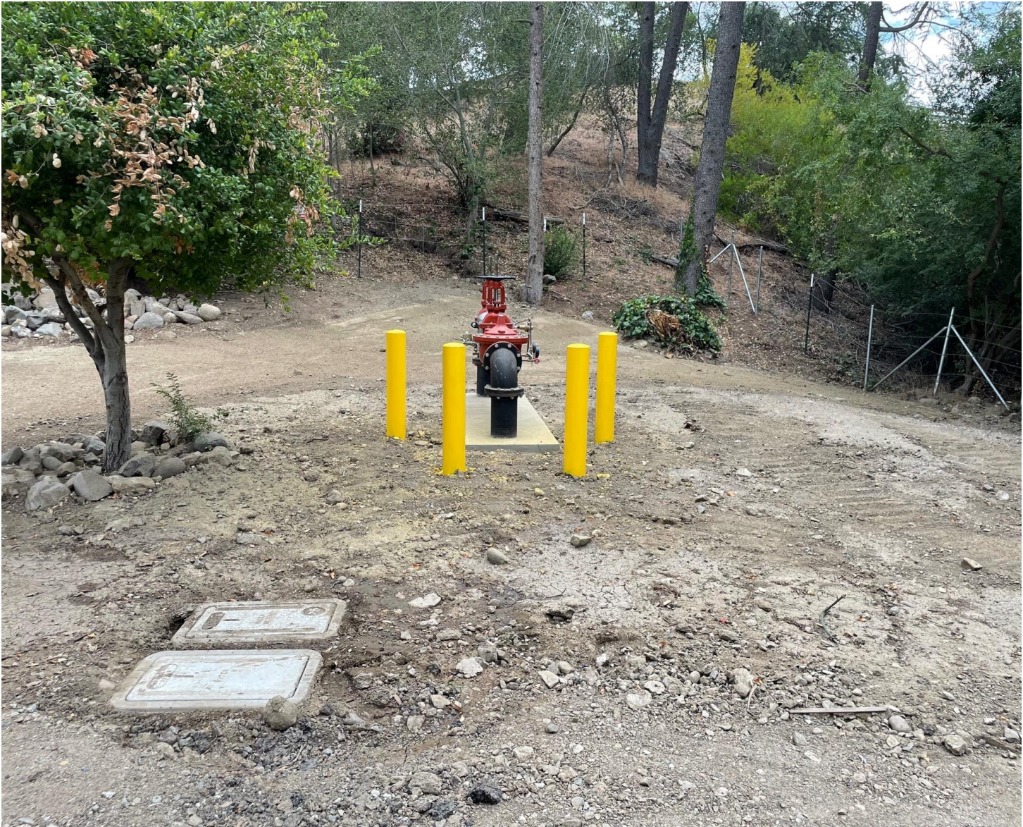
New DCDA and Domestic/Irrigation Meters
