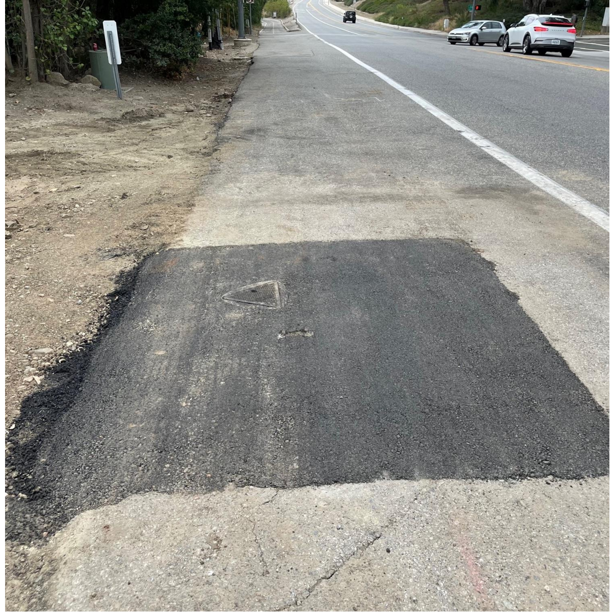
New Valve (Hot Tap) & Paving in El Toro Rd
