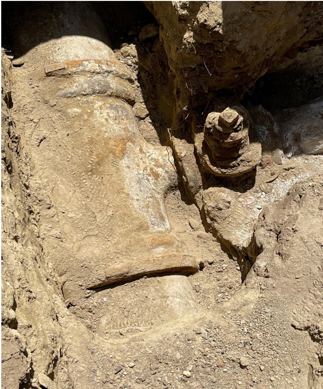
Abandoned Connection inside Pumping Plant Yard & Paving
