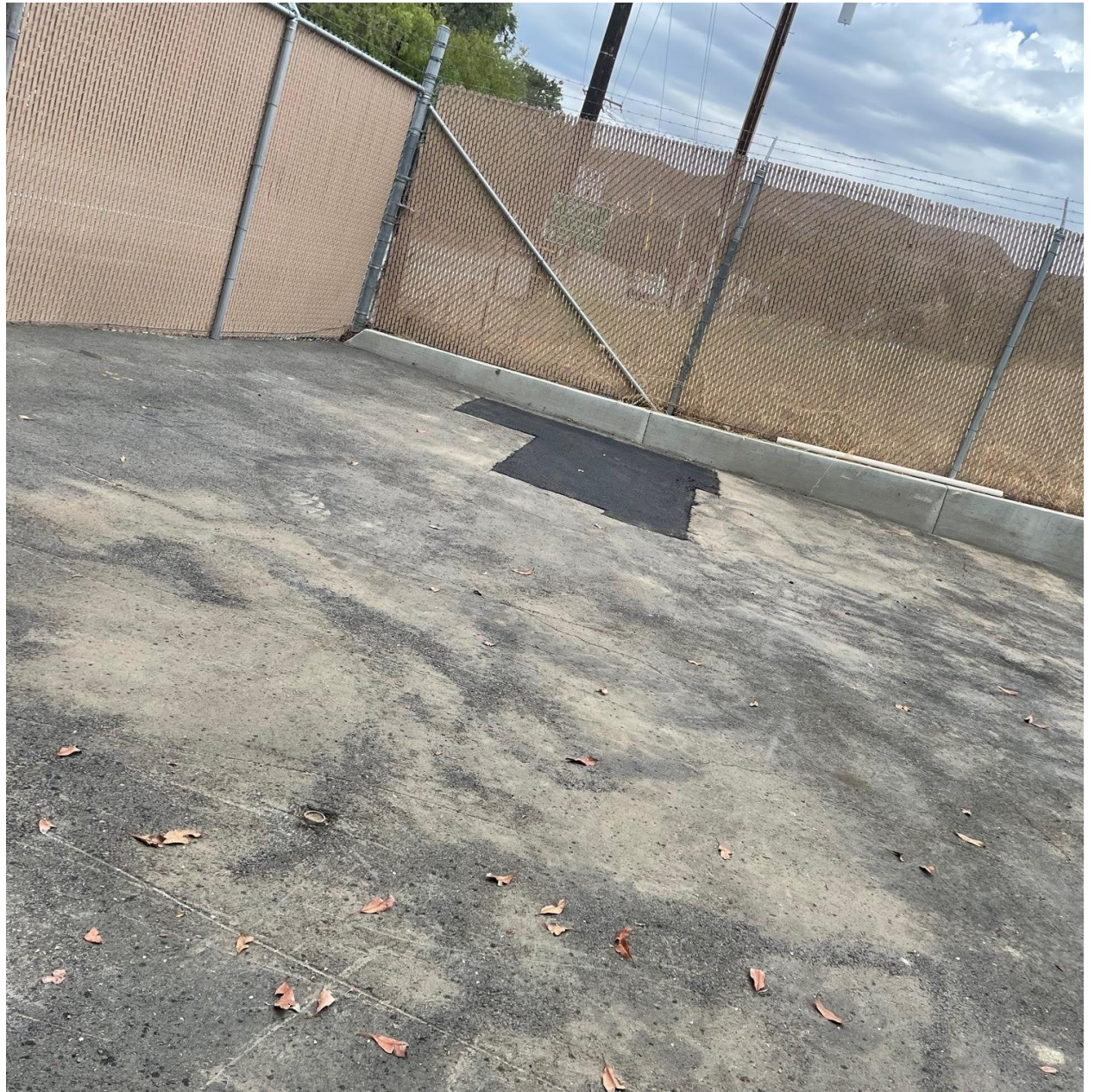
Abandoned Connection inside Pumping Plant Yard & Paving
