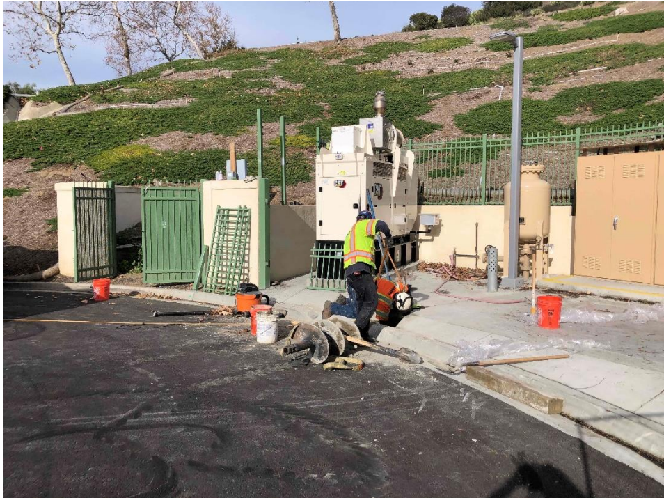
Removing Existing Pole to Deepen Foundation
