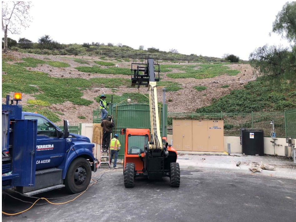
Installation of 10-foot Man Gate
