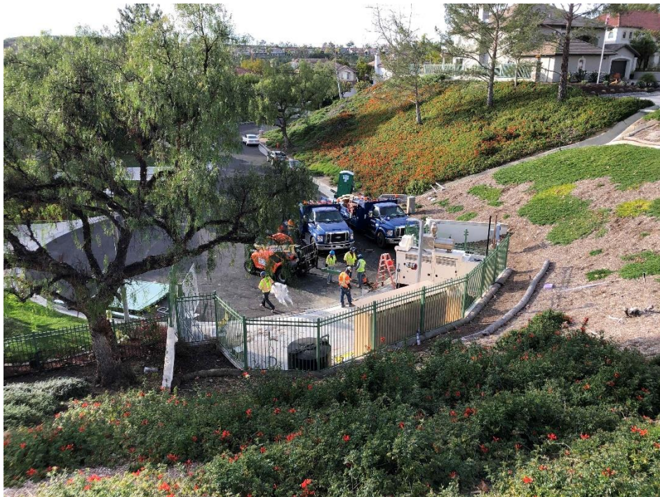
FERREIRA Removing Existing Swing Gates
