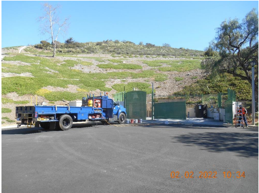
Contractor Final Clean Up of Site
