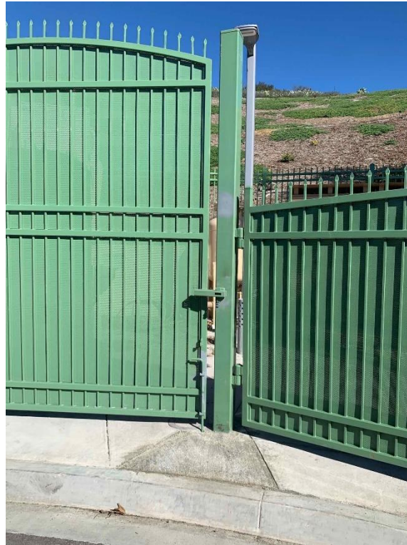
Gates Installed and Post Extended
