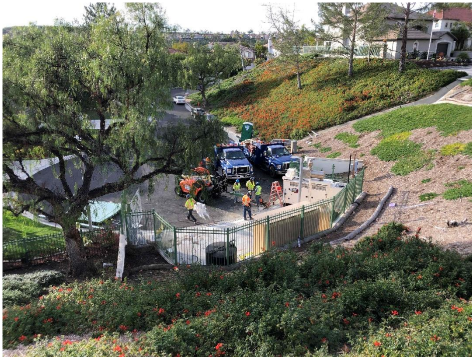
FERREIRA Removing Existing Swing Gates
