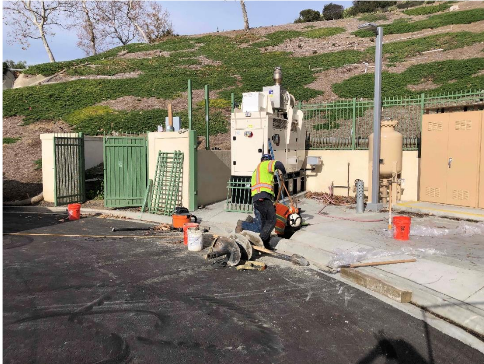
Removing Existing Pole to Deepen Foundation
