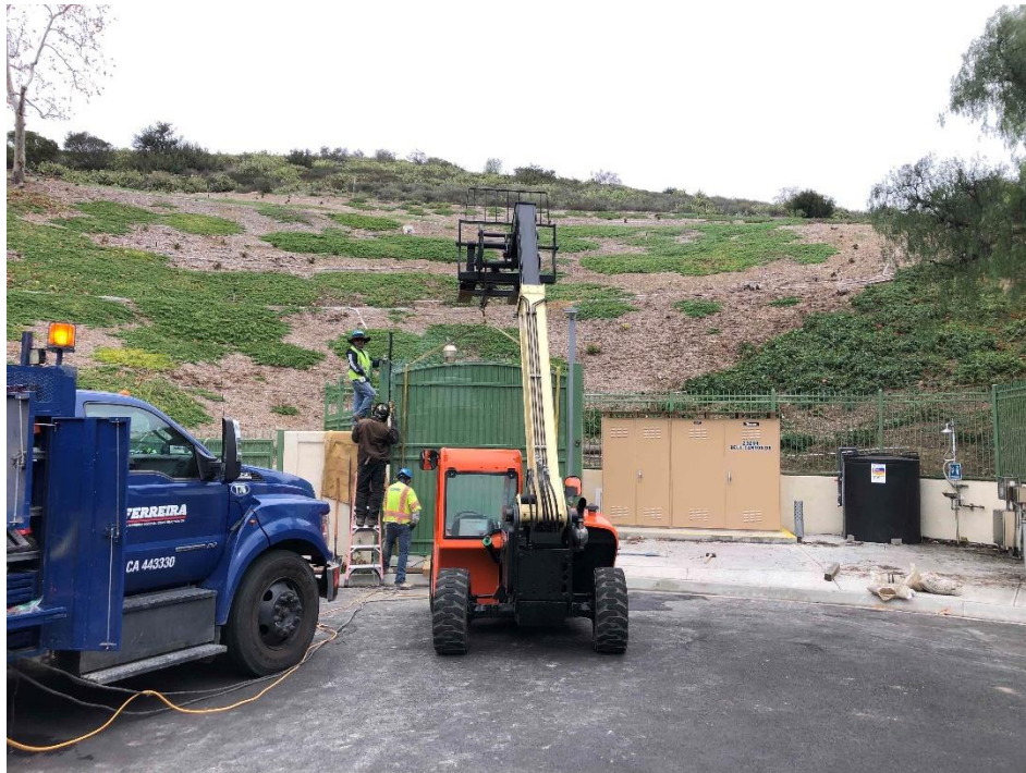
Installation of 10-foot Man Gate
