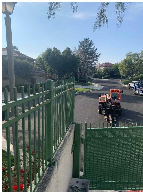
Swing Gates Re-installed with New Perforated Metal Screens
