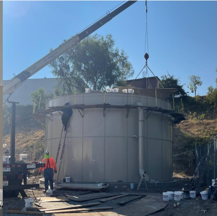
New Tank Exterior During Construction Process
