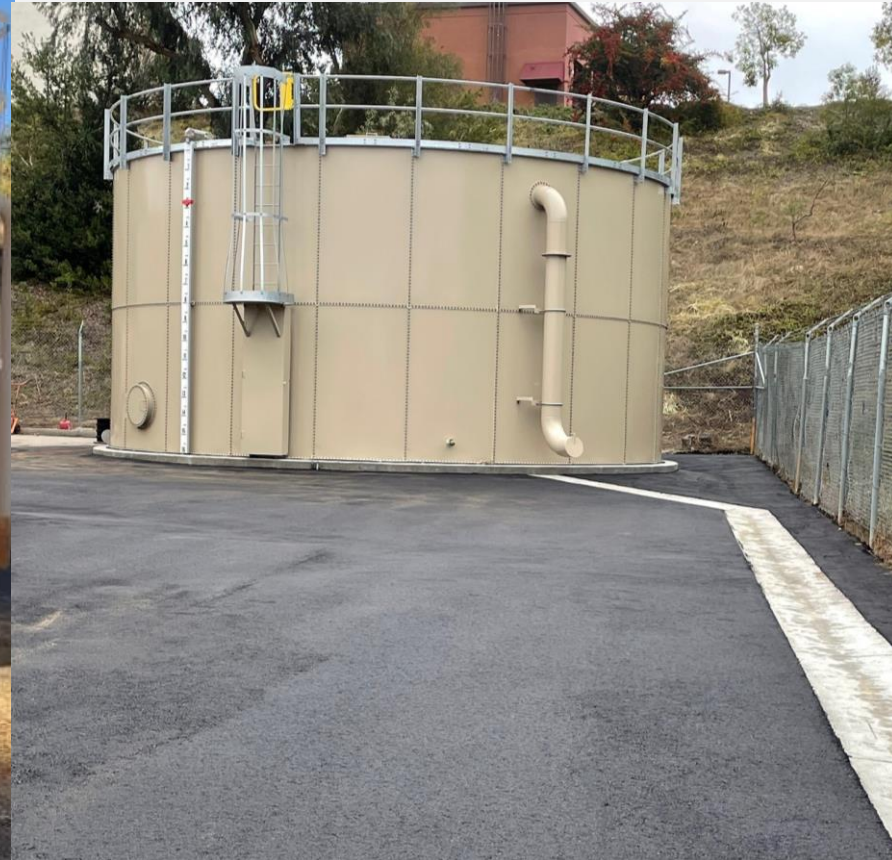
New Tank, Abandonments, Paving and Drainage.
