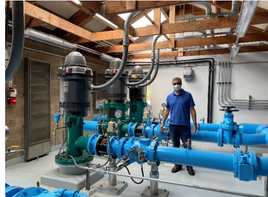
Steve Conner, Engineer of Record for Ridgeline Pump Station
