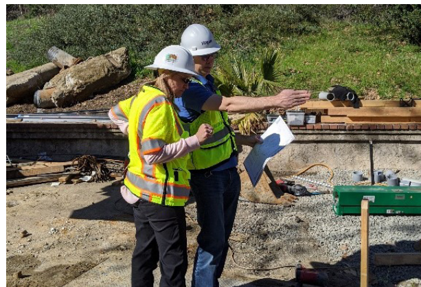
Steve Conner observing construction at Ridgeline Pump Station
