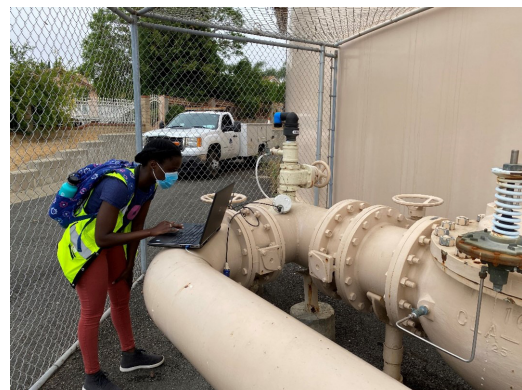
Modeling team member Peace Maari setting up a pressure recorder for model calibration.
