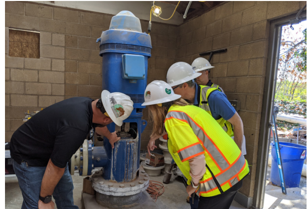
Hazen team examining existing pumps at Ridgeline prior to replacement
