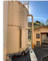
Photo 1 – Existing 42,000-Gallon Backwash Settling Tank
