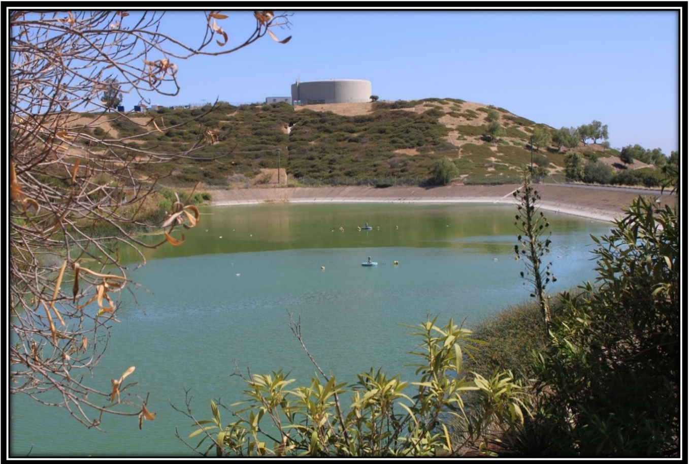
DOVE TANK OVERLOOKING RECYCLED WATER RESERVOIR AT ROBINSON RANCH WASTEWATER TREATMENT PLANT
