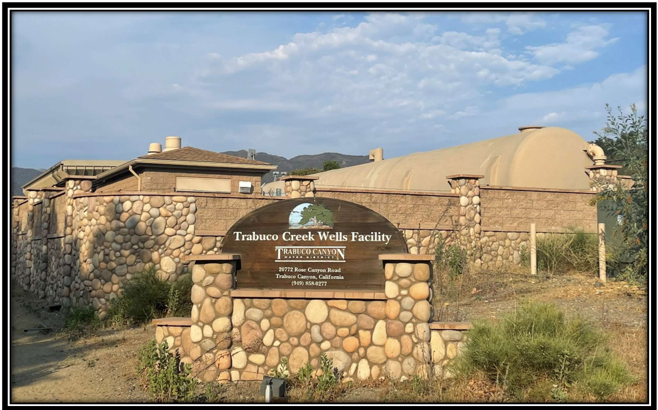
TRABUCO CREEK WELLS FACILITY
