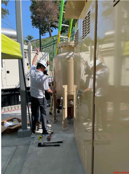
Completing Surge Tank (BLACOH) Install and Testing
