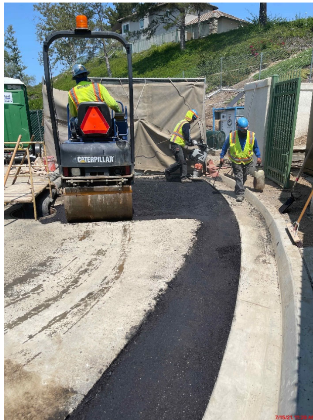
Asphalt Paving Section and Restoration
