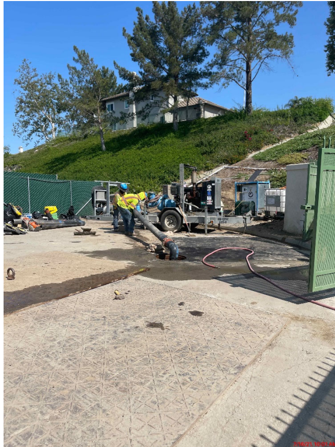
Removal of Temporary Sewer By-Pass System and Temporary Fencing
