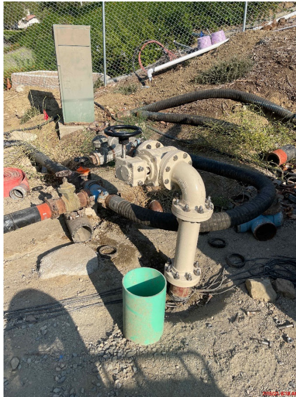
Install Plug Valve for Aboveground Bypass Section
