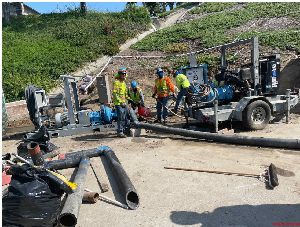
Removal of Temporary Sewer By-Pass System and Temporary Fencing
