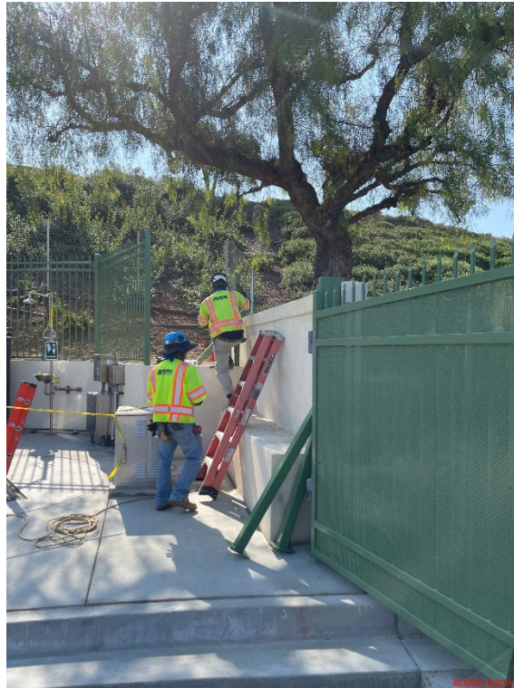
Install Additional Wrought Iron Fencing
