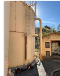
Photo 1 – Existing 42,000-Gallon Backwash Settling Tank
