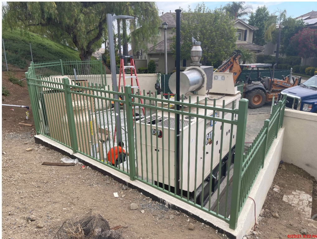
Wrought Iron Fencing Installed
