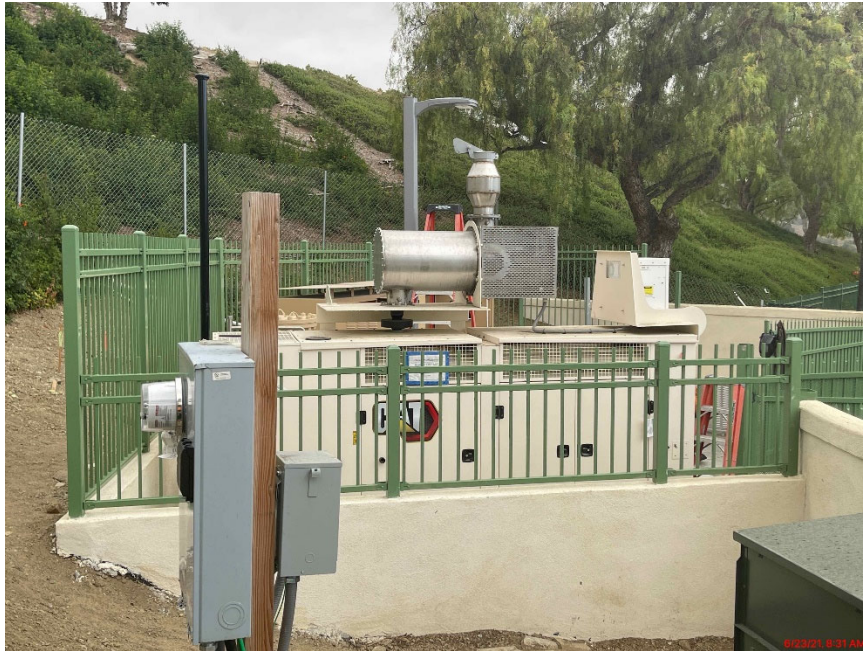
Wrought Iron Fencing Installed
