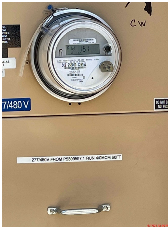
SCE Meter Installed and Lift Station Energized
