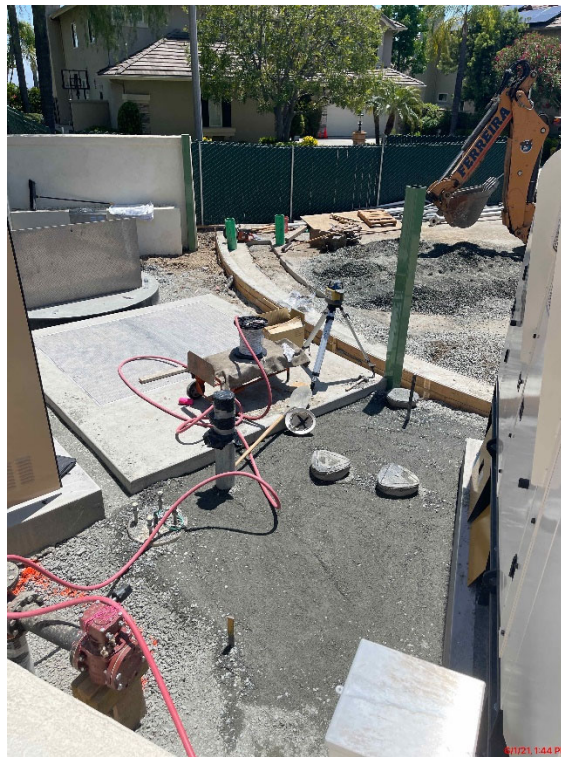
Base Paving for Sidewalk Areas
