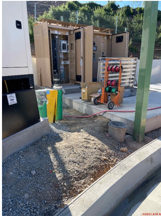
Continuing with wiring in MCC Panel
