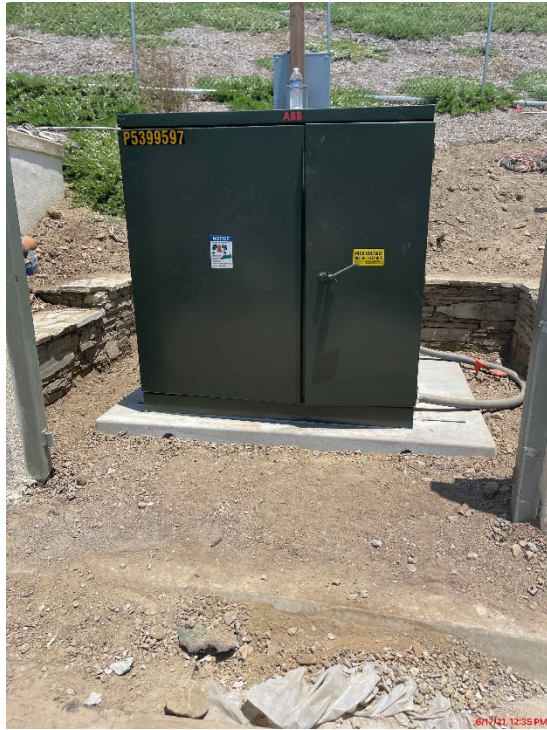
New Transformer Installed
