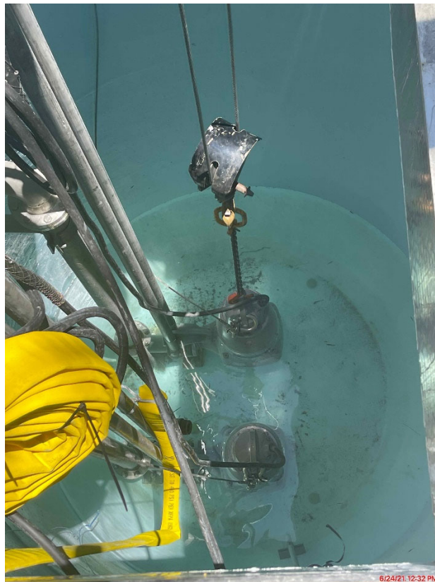
Pumps Submerged and Tested
