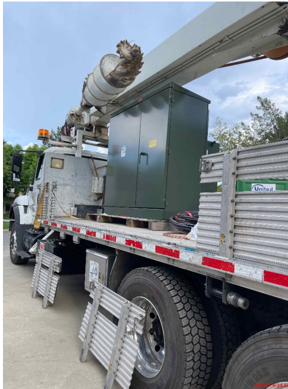
SCE Transformer Delivered to Lift Station
