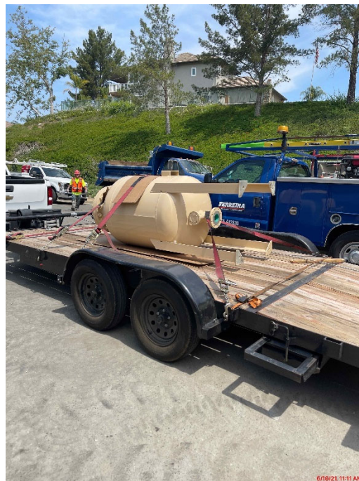
Surge Tank Delivered to Lift Station
