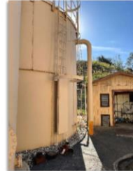
Photo 1 – Existing 42,000-Gallon Backwash Settling Tank
