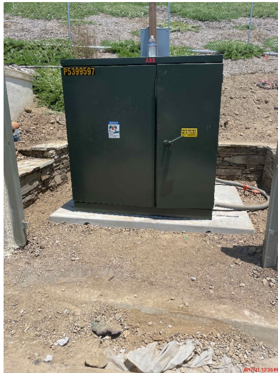
New Transformer Installed
