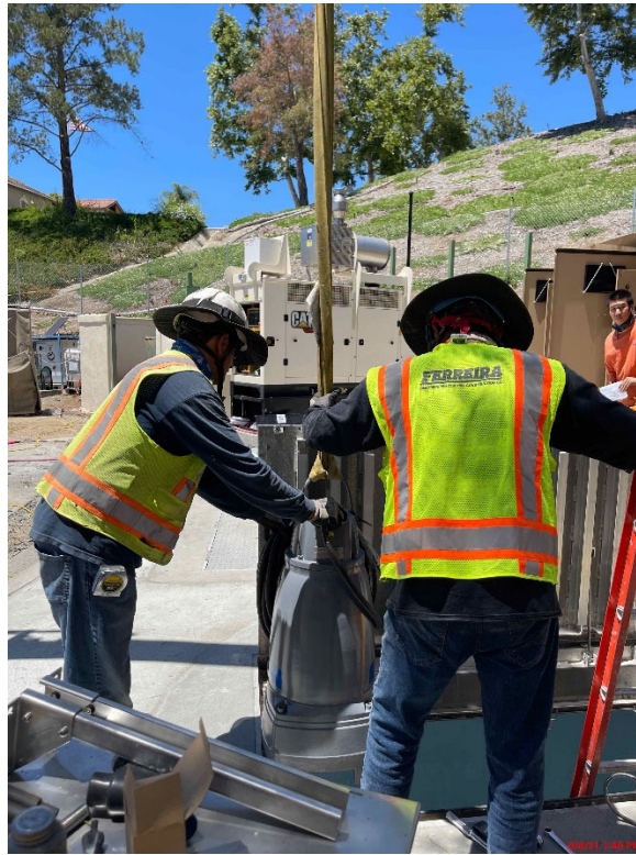
Placement of Pumps
