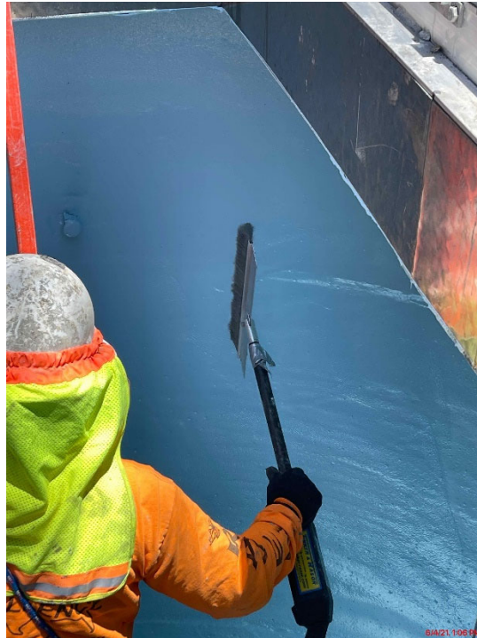
Coating of Wet Well
