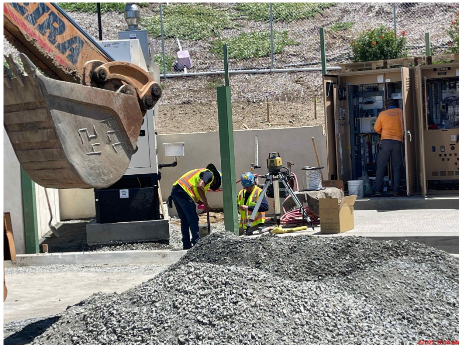
Base Paving of Sidewalk Areas
