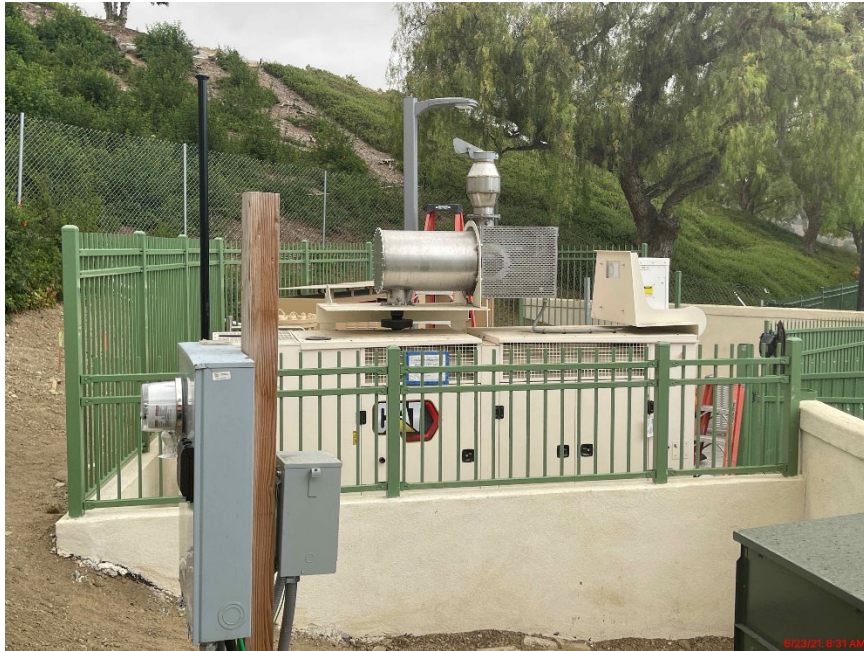
Wrought Iron Fencing Installed
