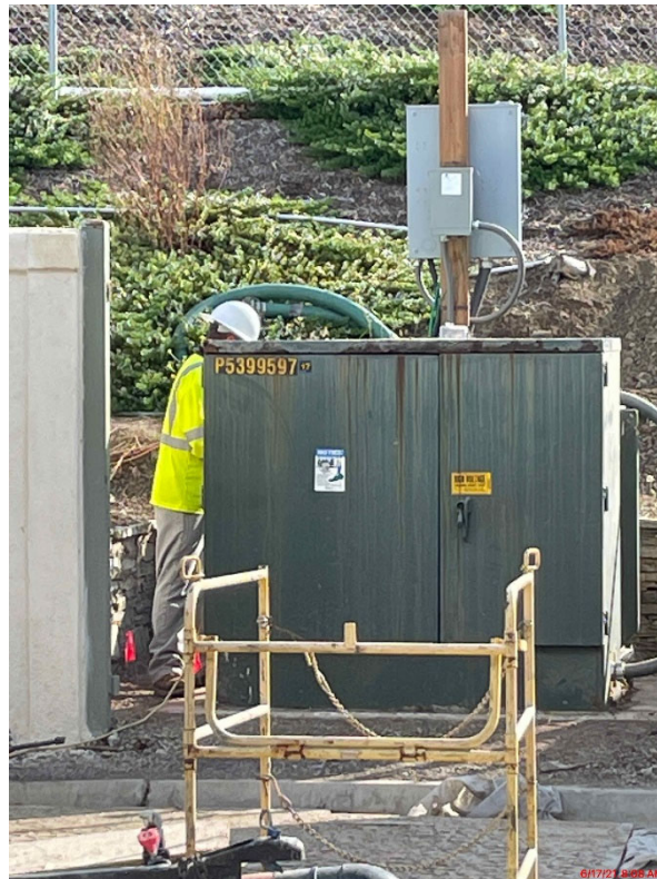
Former Transformer being disconnected and removed
