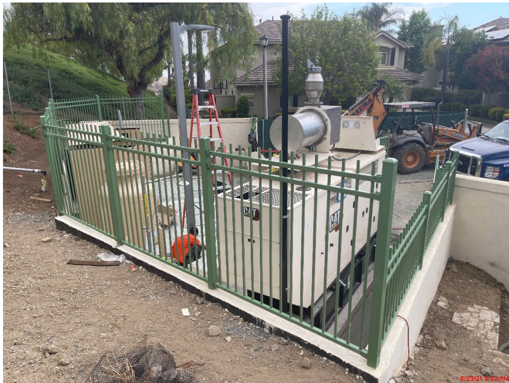
Wrought Iron Fencing Installed
