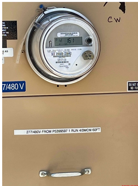
SCE Meter Installed and Lift Station Energized
