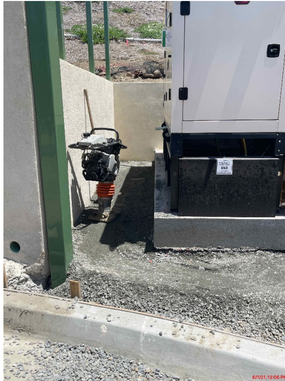
Base Paving for Sidewalk Areas
