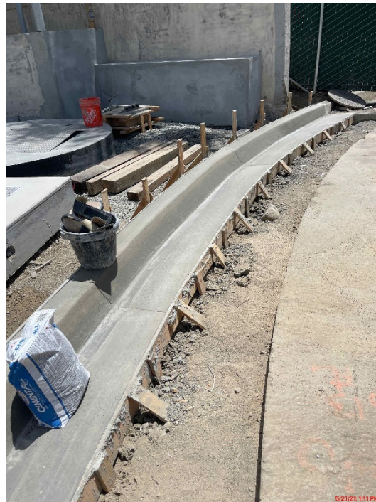
Poured Rolled (or Mountable) Curb
