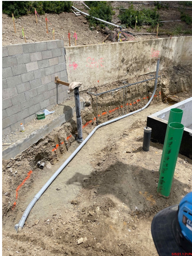
Placement and extension of new, 3-inch SCE Conduit
