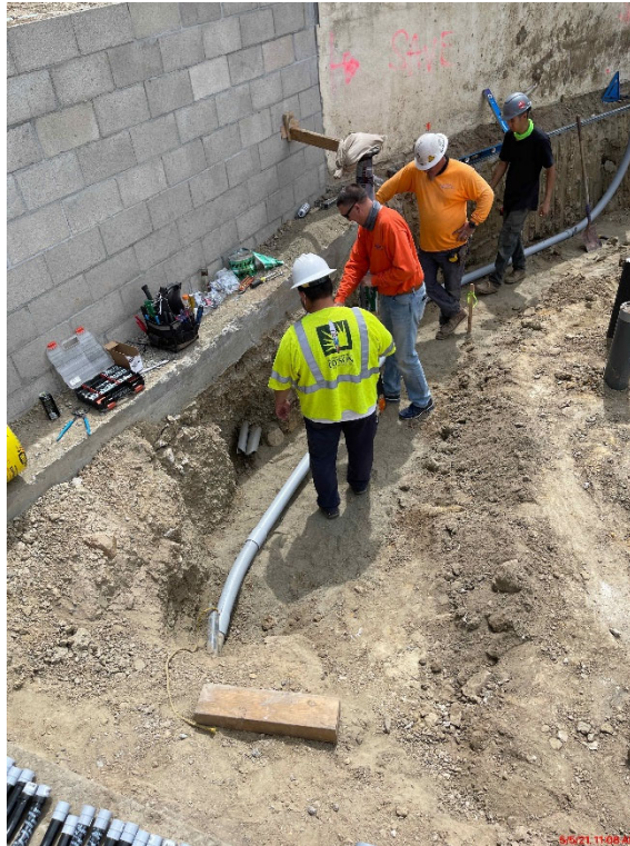
SCE Inspection of new and extended SCE conduit
