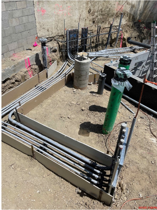
Forms for electrical duct bank
