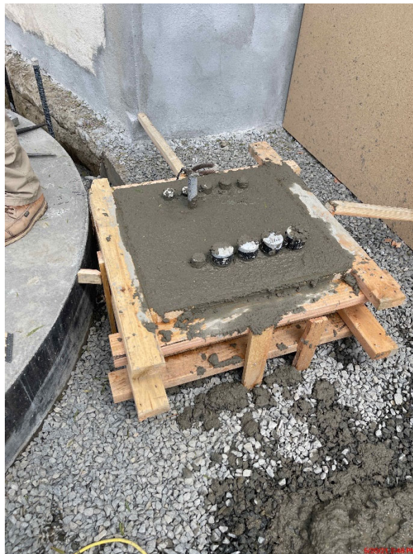
Poured Sump Termination Pad
