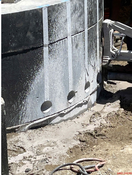
Coring into Wet Well for electrical penetrations
