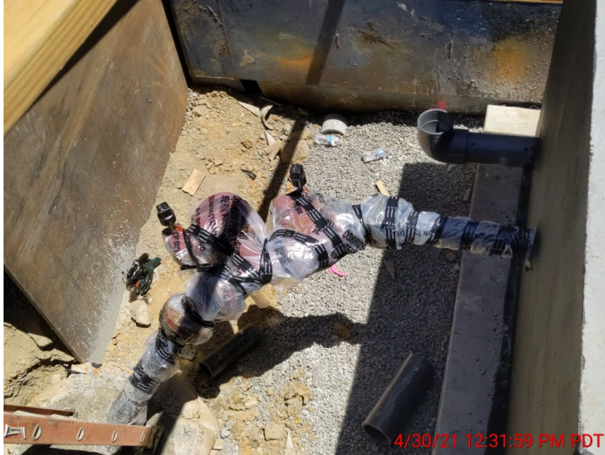
Wrapping Mechanical Piping for direct burial during backfill
