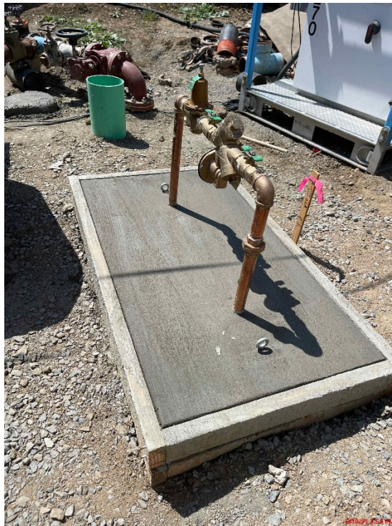
Installed new backflow device and cage
