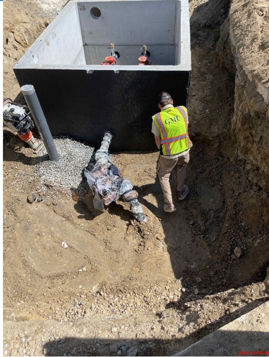
GMU inspecting backfill placement
