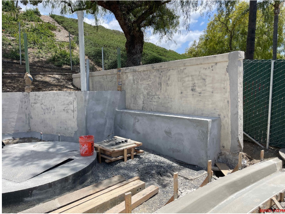
Stucco preparation of new and existing Walls
