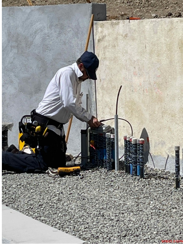
AT&T representative extending wire and restoring service to new MCC Panel
