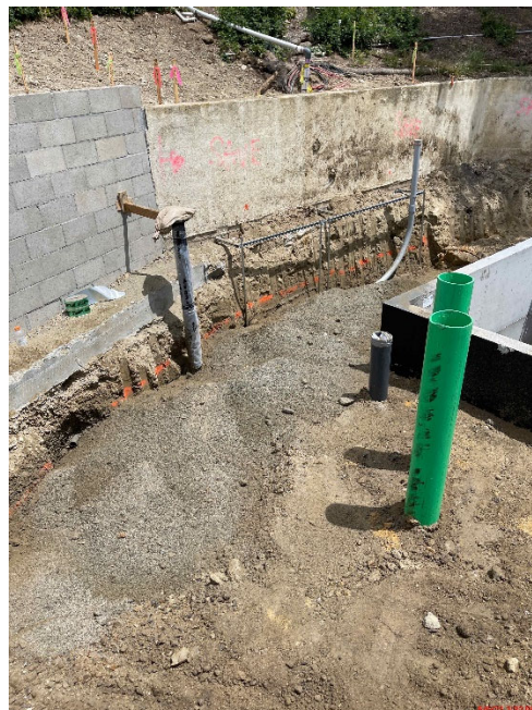
Upon completion of SCE Inspection, SCE conduit backfilled
