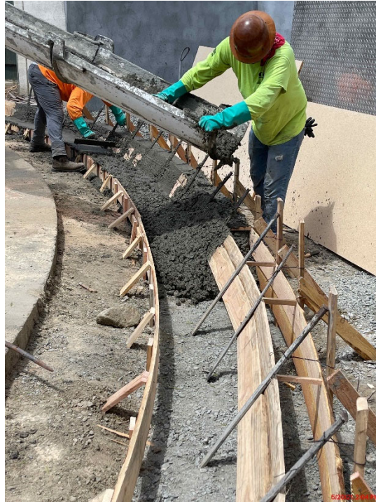
Form and pour Rolled (or Mountable) Curb
