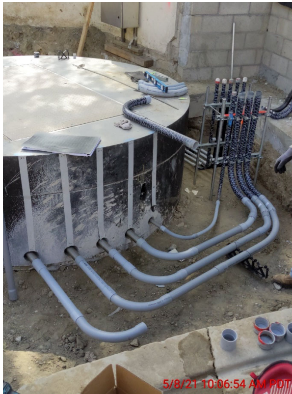
Setting Wet Well
