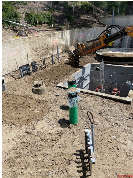
Backfill electrical duct bank
