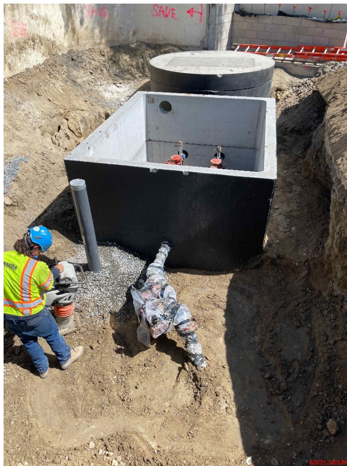
Backfill of Mechanical Piping
