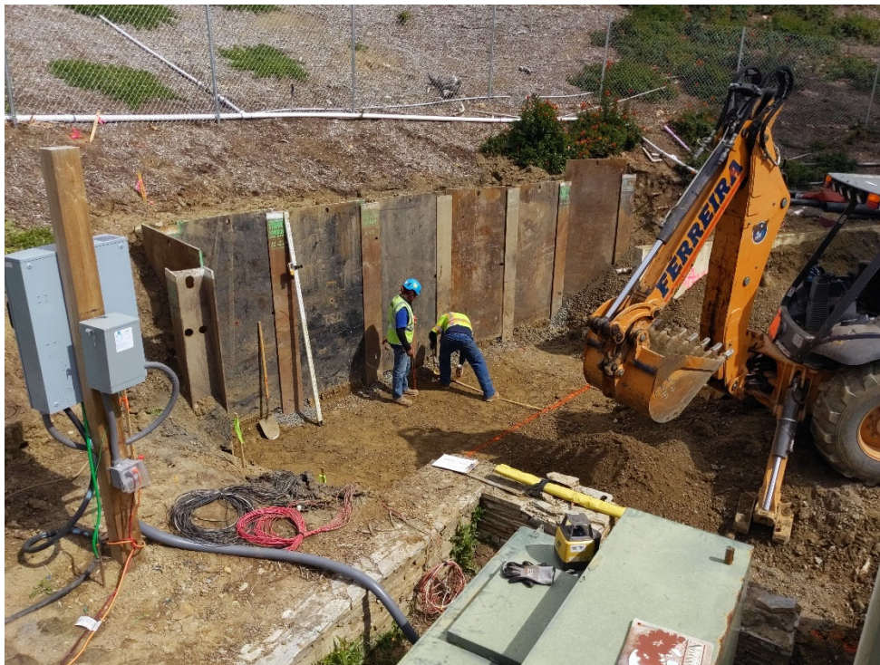
Making subgrade (or bottoms) of Wall Footings and Shoring Completed
