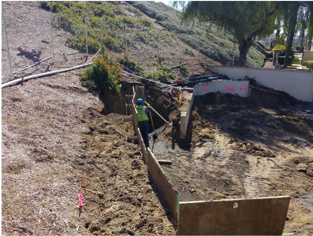
View of Shoring System
