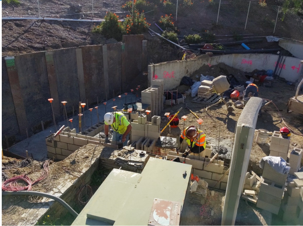
Delivery and installation of Masonry Block Wall
