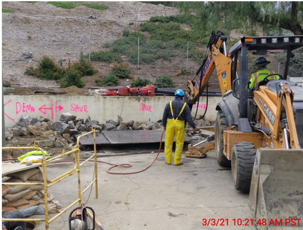
Demolition Efforts of Lift Station
