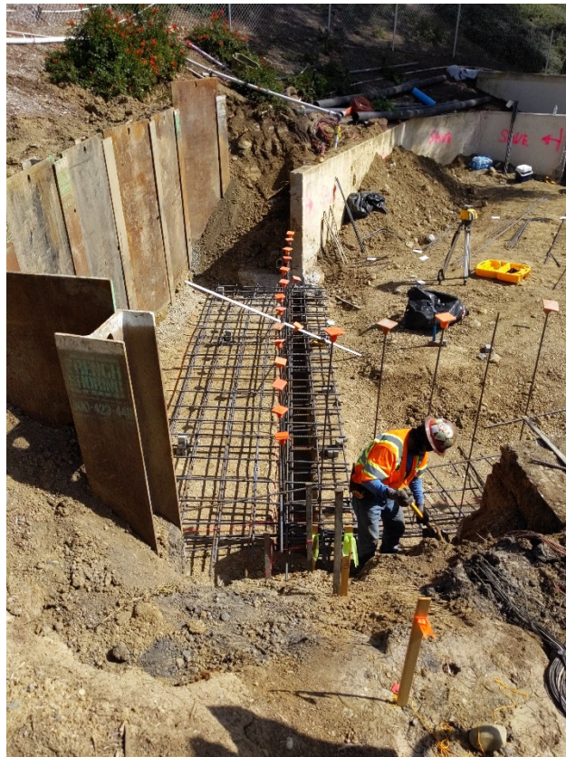
Placement of steel reinforcement bars and forms for Wall Footings
