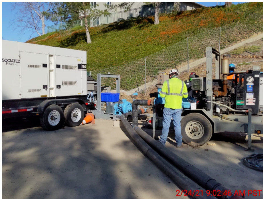
Rain-for-Rent delivered and installed Sewer By-Pass System
