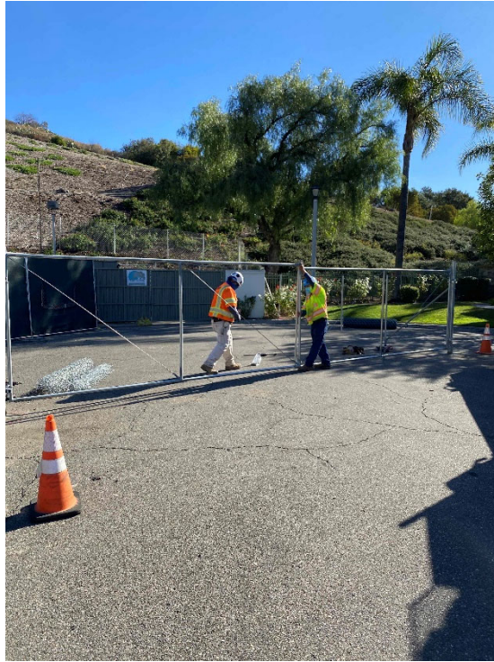
Installing Temporary Fence Enclosure to protect Project
