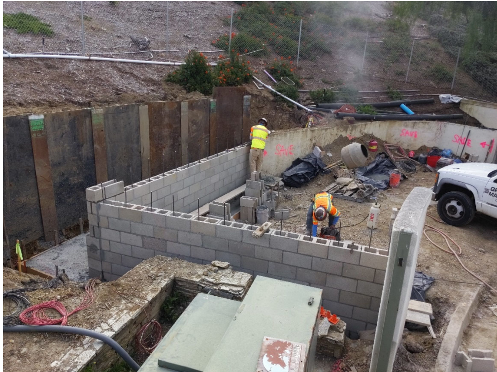
Continuing installation of Masonry Block Wall
