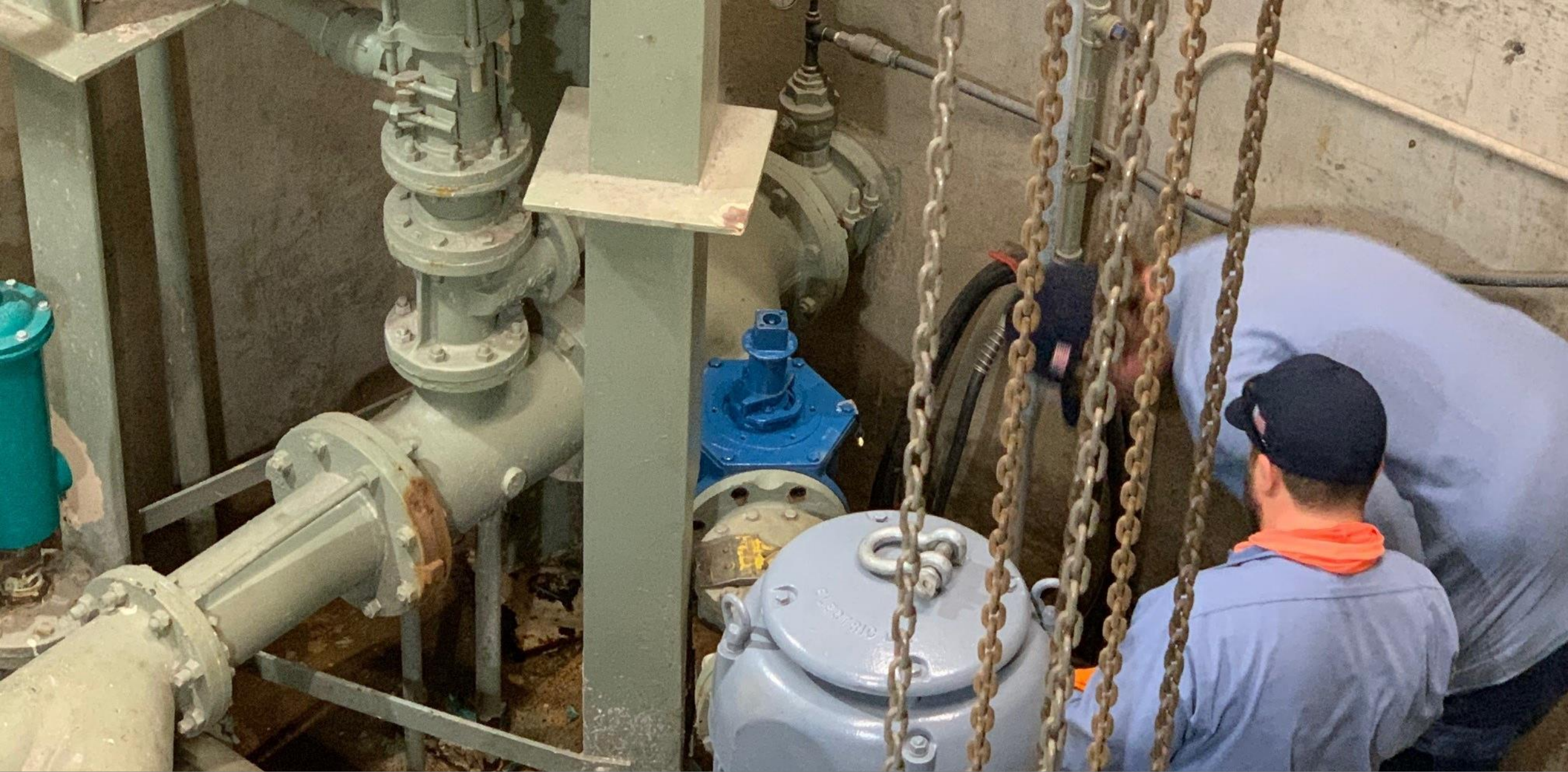
Installation of new Plug Valve (Blue) in station dry pit.
