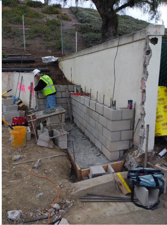
Grout Placement in Masonry Block Walls
