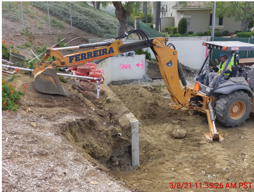
Excavation for Shoring (Vertical) Beam-and-Plate
