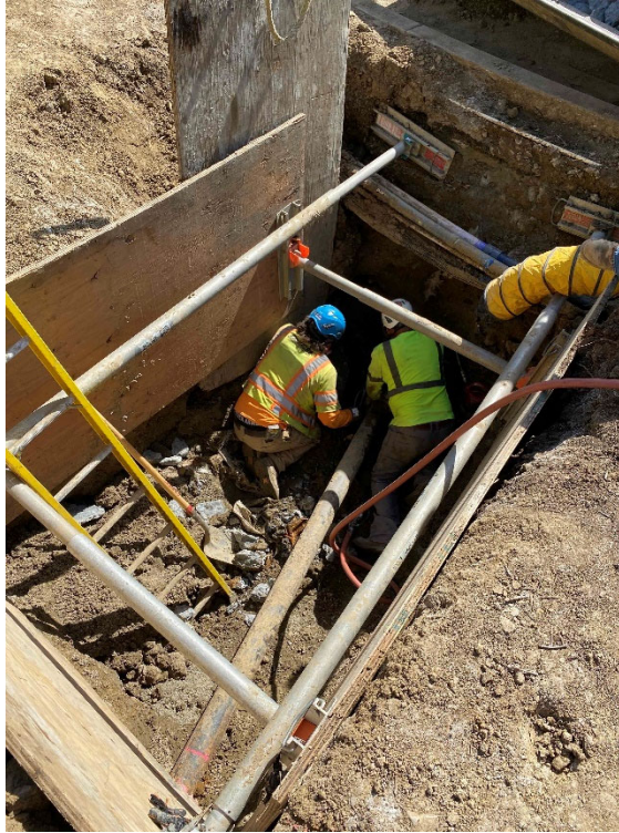
Exposed 4-inch Sewer Force Main for “Cut-In Valve”
