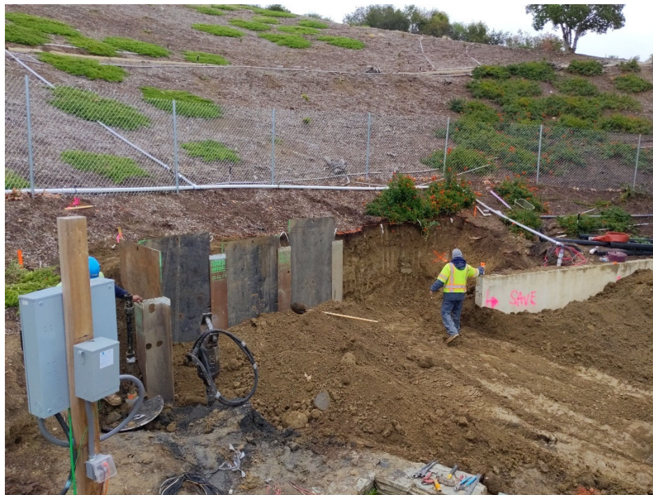
Shoring (Vertical) Beam-and-Plate
