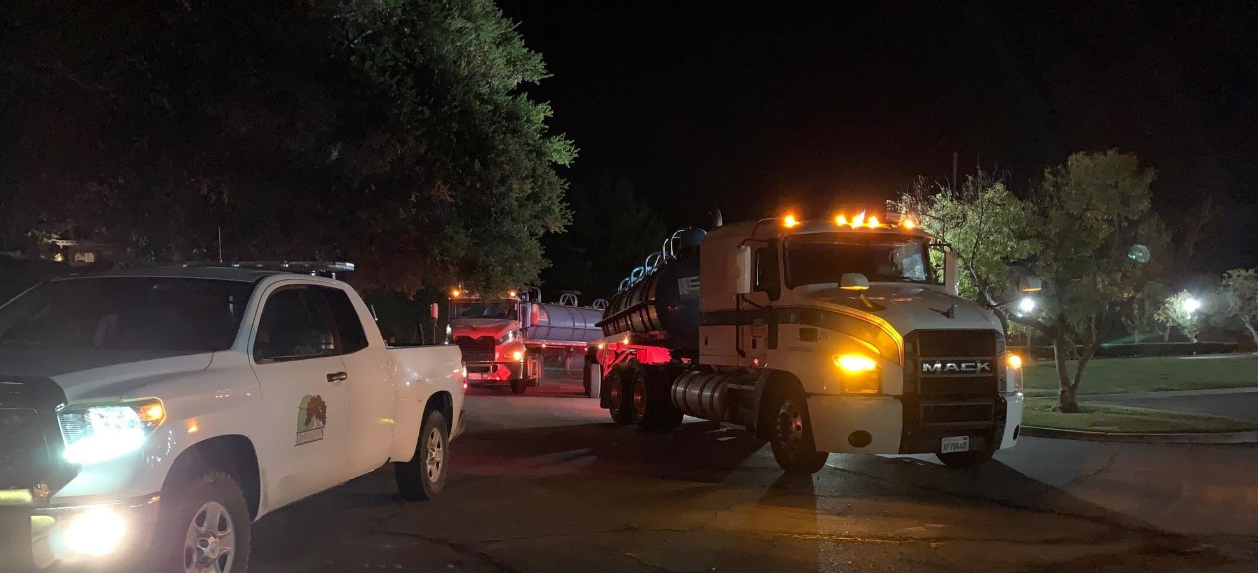
GCSLS PLUG/CHECK VALVE REPLACEMENT JOB MARCH 4, 2021
