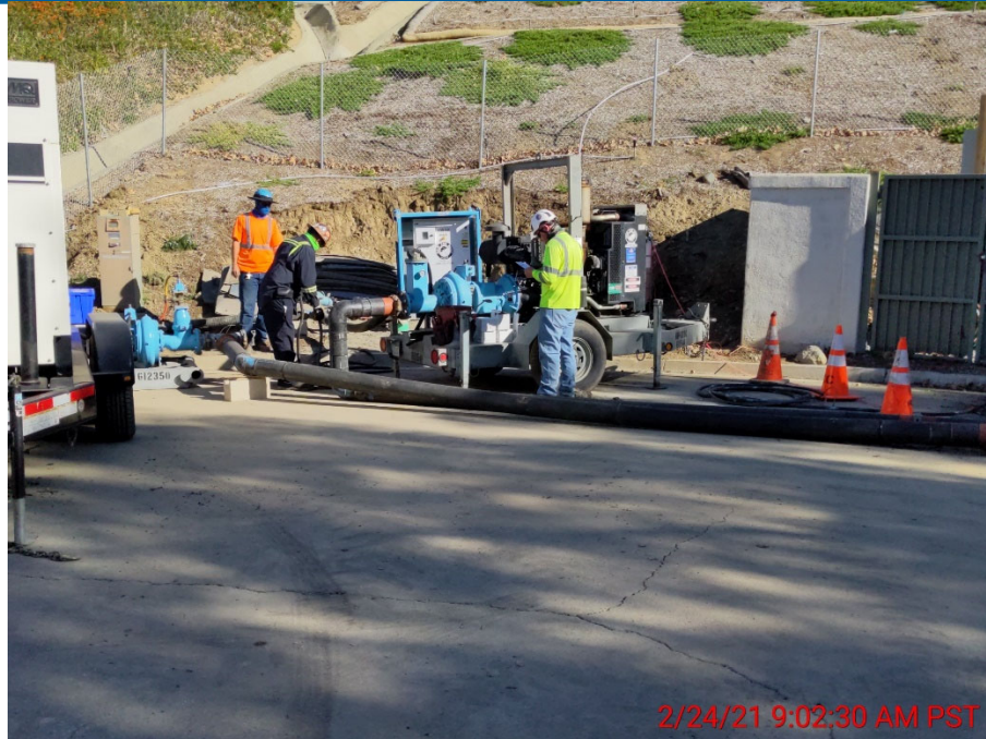
Rain-for-Rent delivered and installed Sewer By-Pass System
