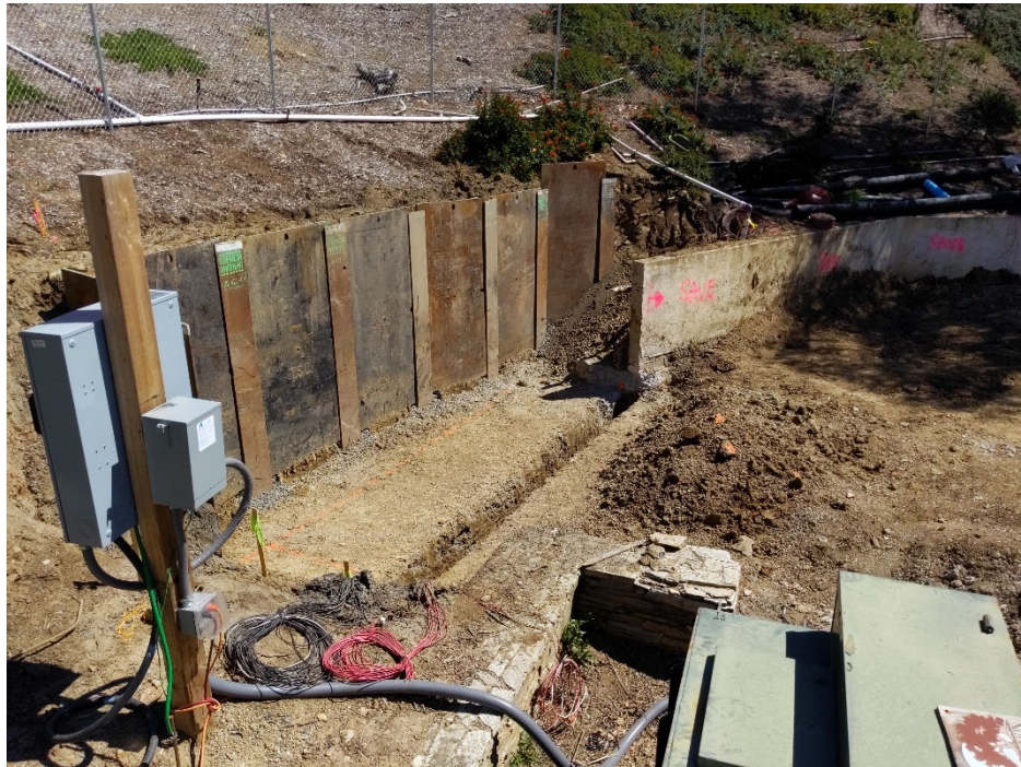
Preparing subgrade and keyway of Footings
