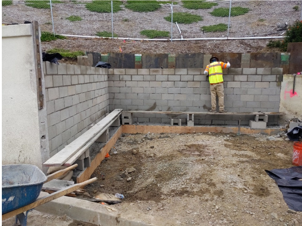
Completing Grout Placement of Masonry Block Walls
