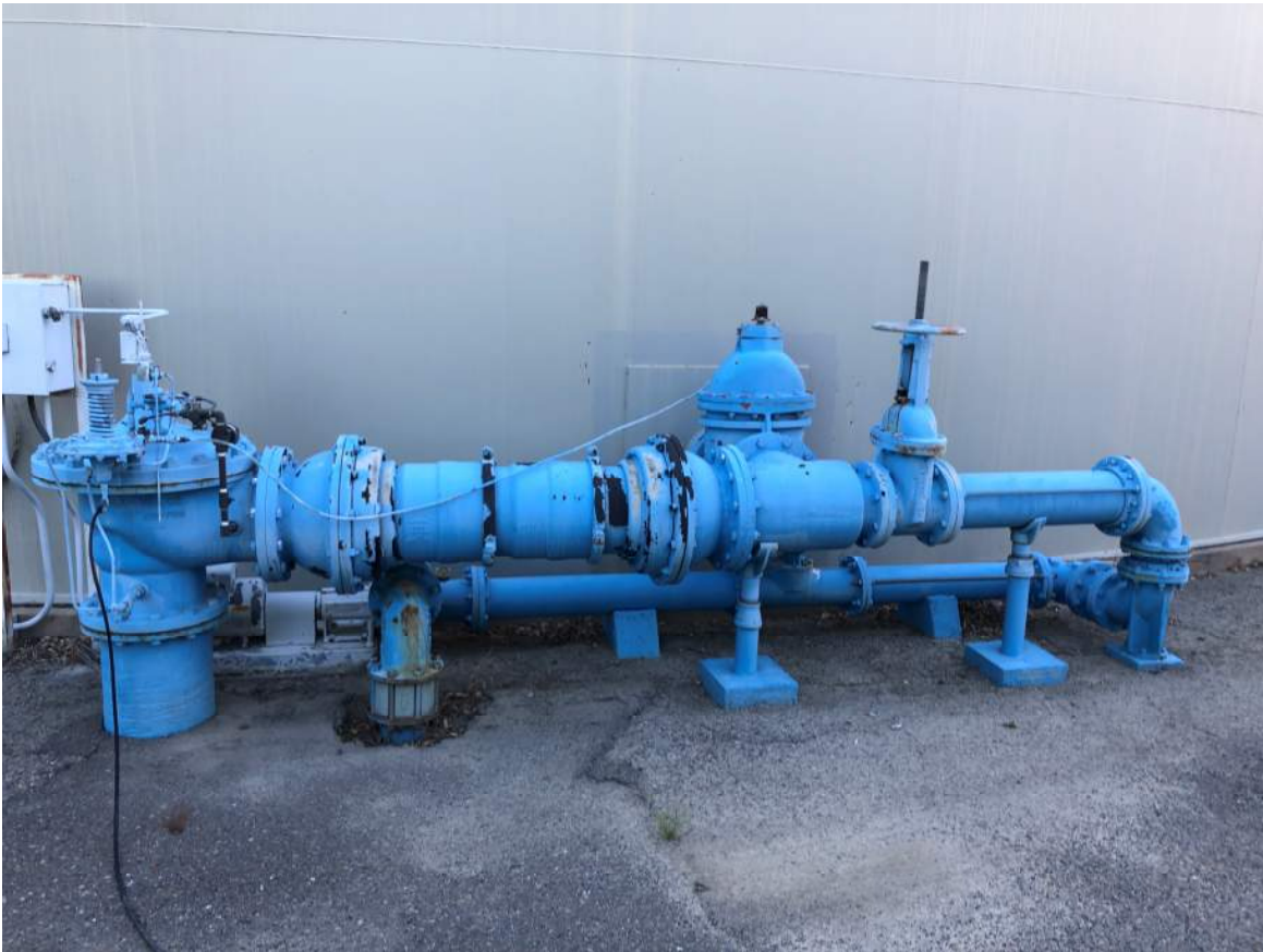
Photo 1 – Existing Reservoir No. 1 Inlet Piping Modification
