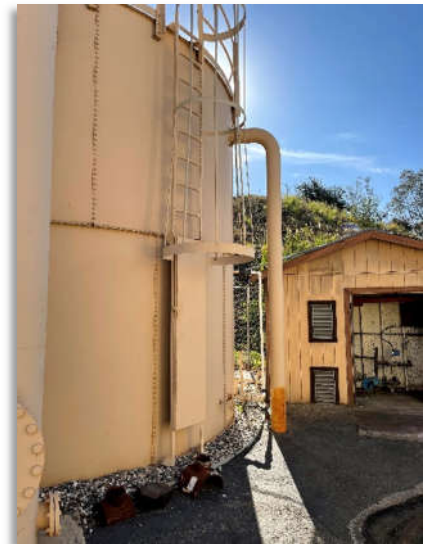
Photo 1 – Existing 42,000-Gallon Backwash Settling Tank
