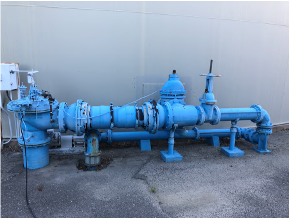
Photo 1 – Existing Reservoir No. 1 Inlet Piping Modification
